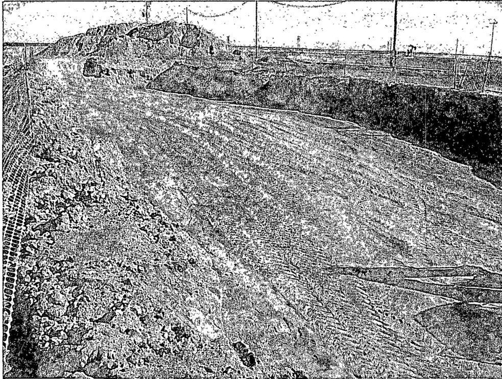
The lower liner was set at an average depth of five feet below ground surface.
