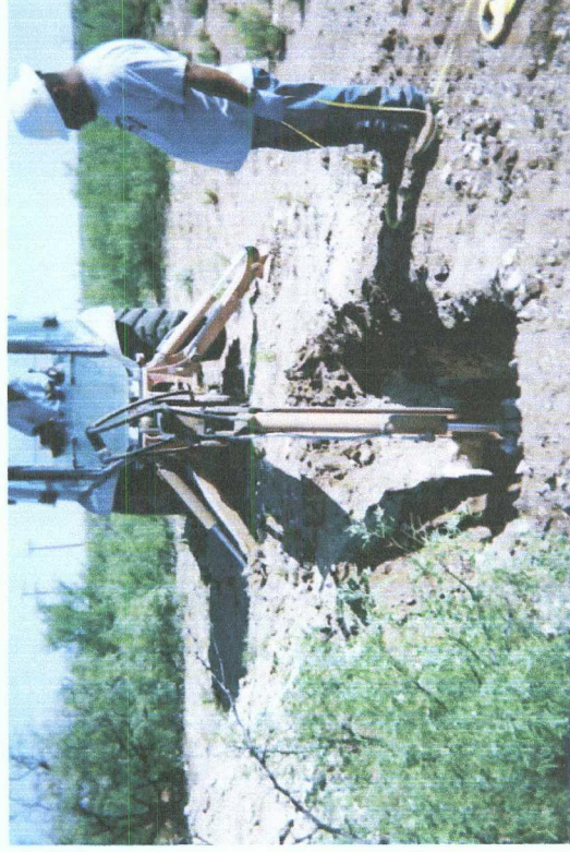
DELINEATION TRENCH BEING EXCAVATED
