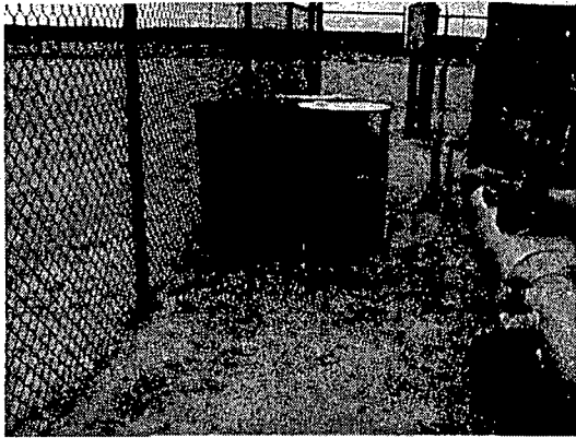
Drums of ethylene glycol stored on ground need to be on impermeable pad
