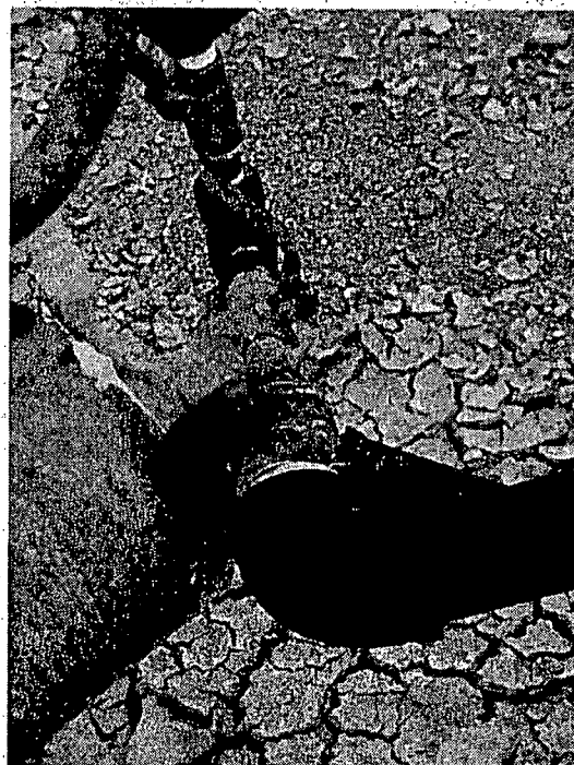
Recommended AFE to replace 1/2 inch dia. pipe with 1 inch or greater.
