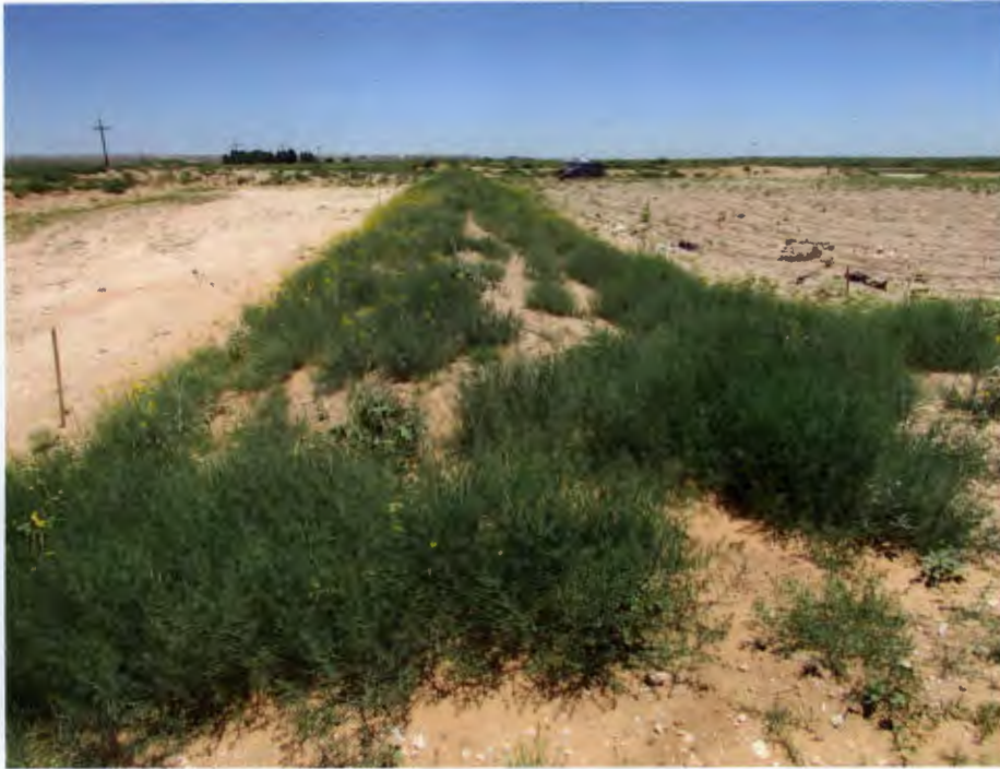
Cell Berm (Cell 1) Viewing East
