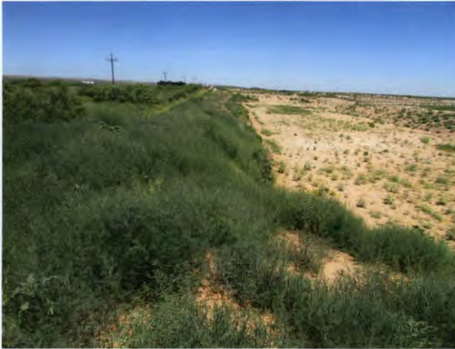
Perimeter Berm (Cell 3) Viewing East
