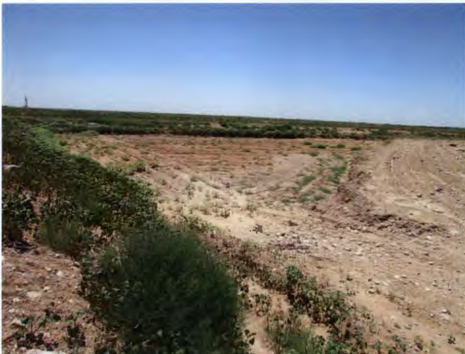
Cell 5 (Southeast Corner) Excavation Viewing Northwest
