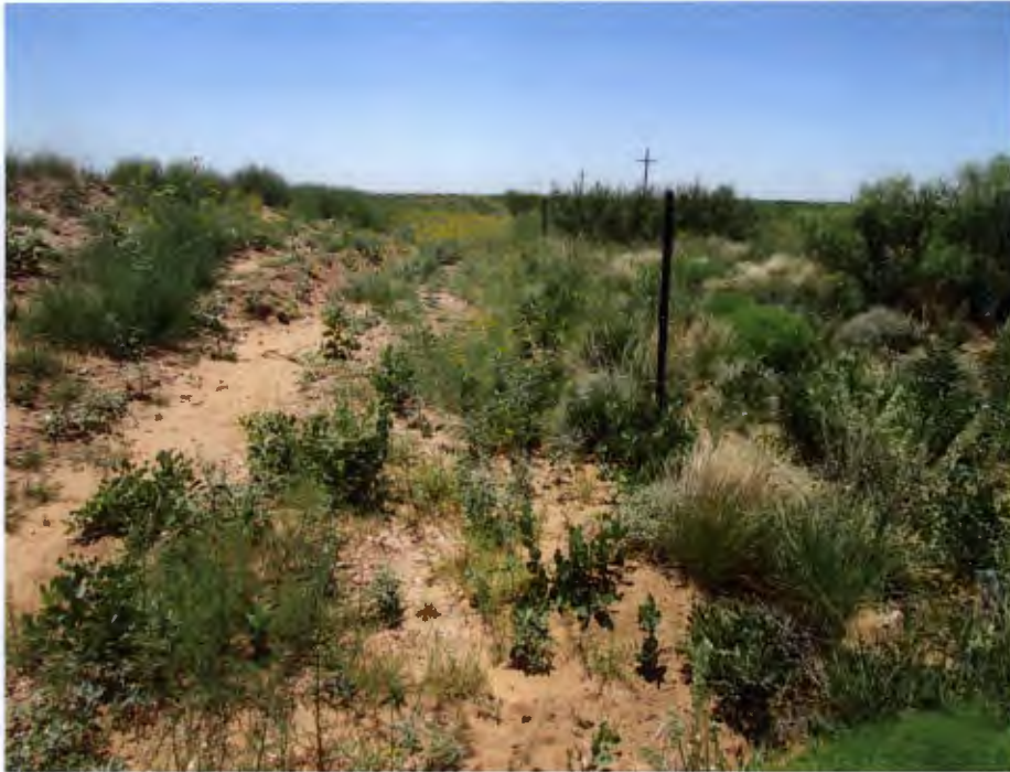
Perimeter Berm and Fence (Cell 1) Viewing West
