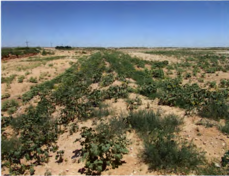
Cell Berm (Cell 3) Viewing East
