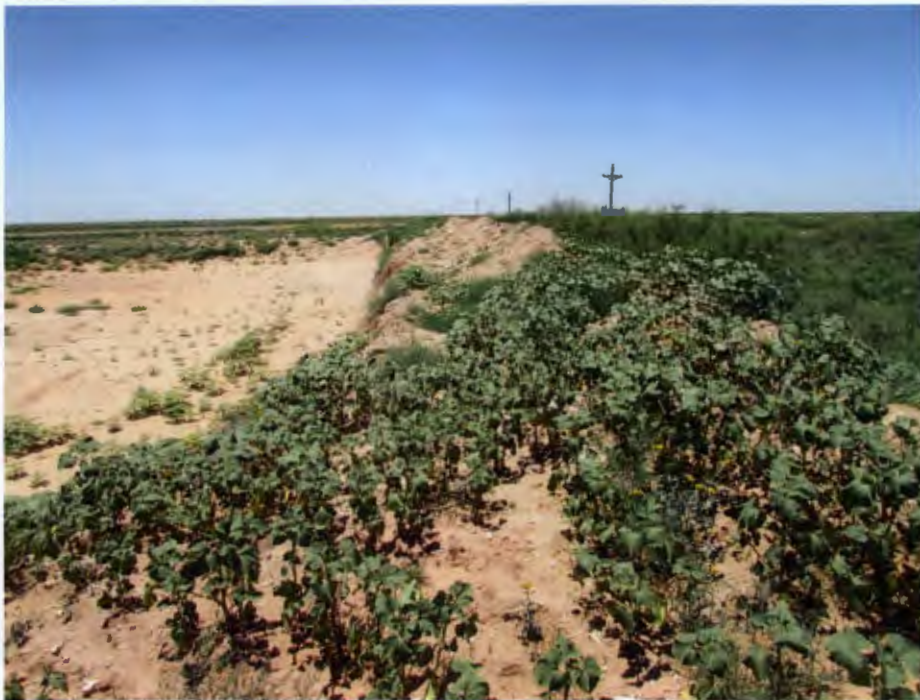
Perimeter Berm (Cell 2) Viewing West
