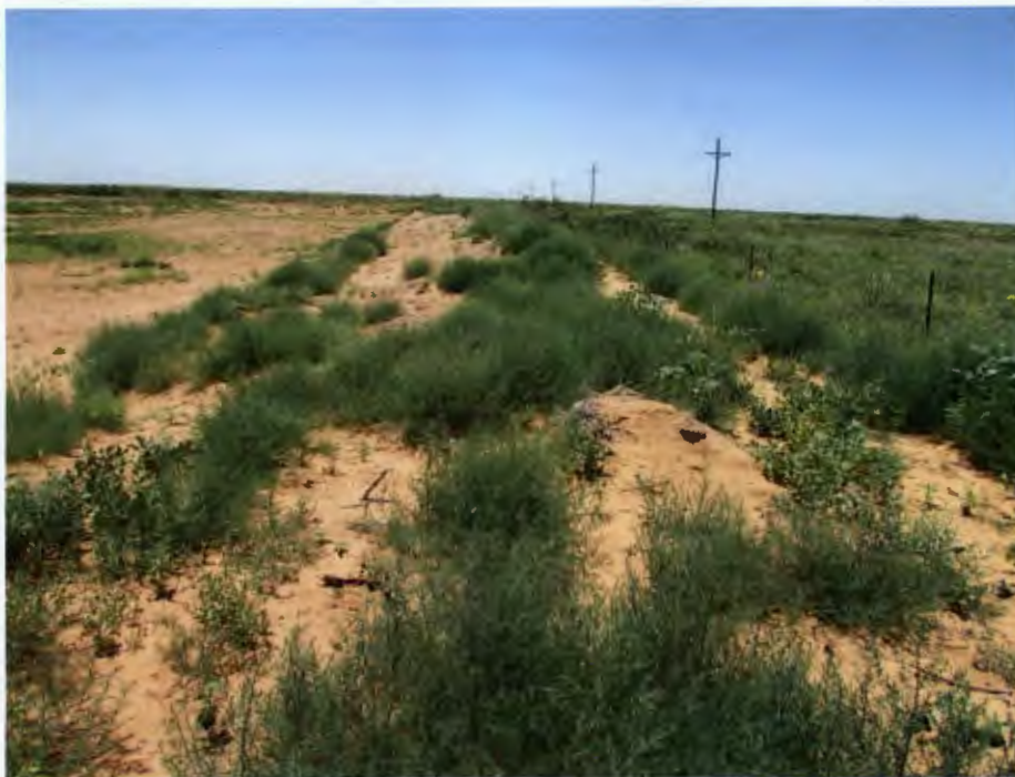
Perimeter Berm (Cell 4) Viewing West
