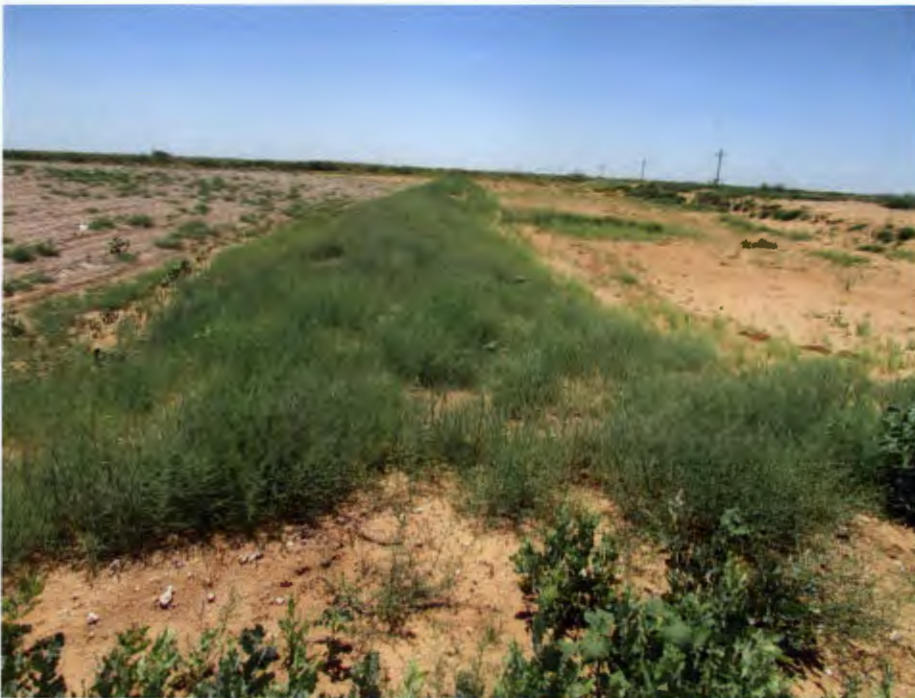
Cell Berm (Cell 4) Viewing West
