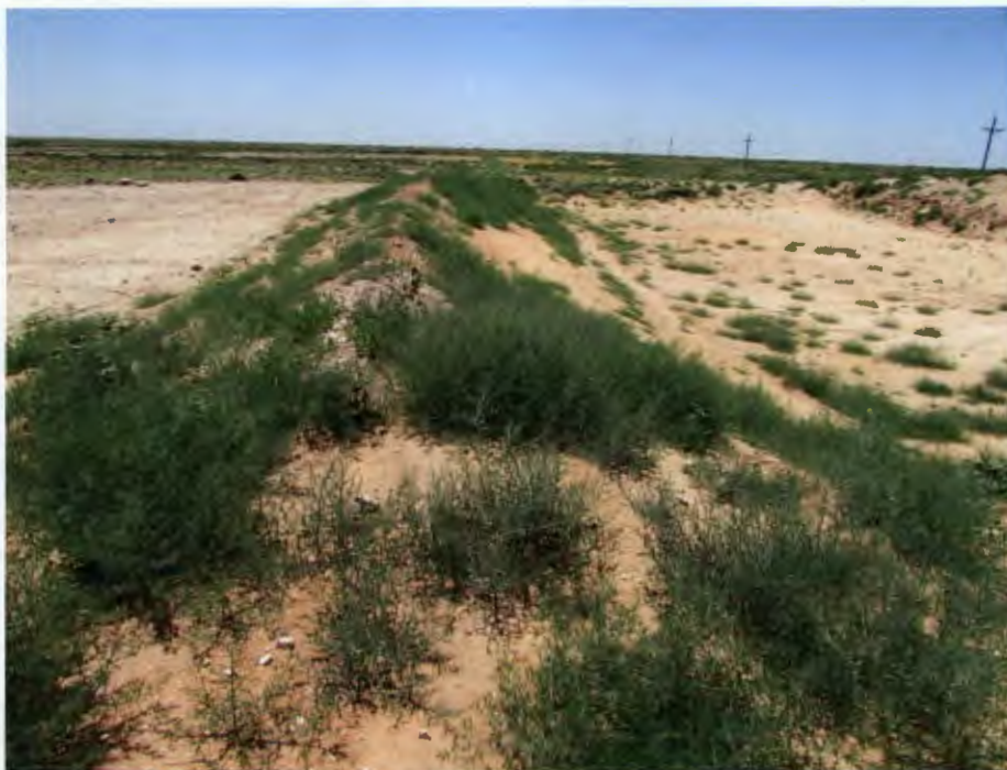
Cell Berm (Cell 2) Viewing West
