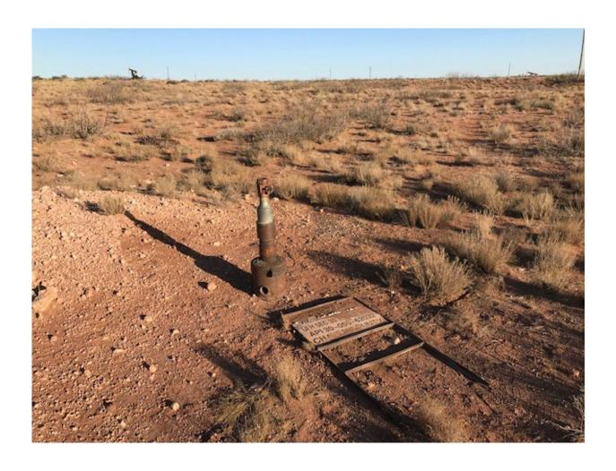
Plains #29-4 (30-005-61904). No rods or valve on tubing (2 photos).
