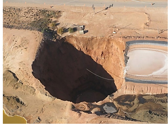
Loco Hills Water Disposal (11/2008)
