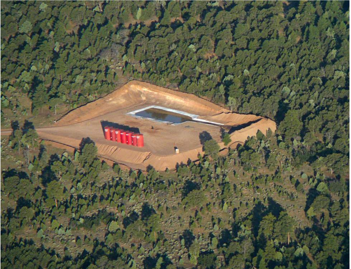
An oil and/or gas site in Aztec, New Mexico, Sept. 2008. Photo credit: Jane Pargiter, EcoFlight.
