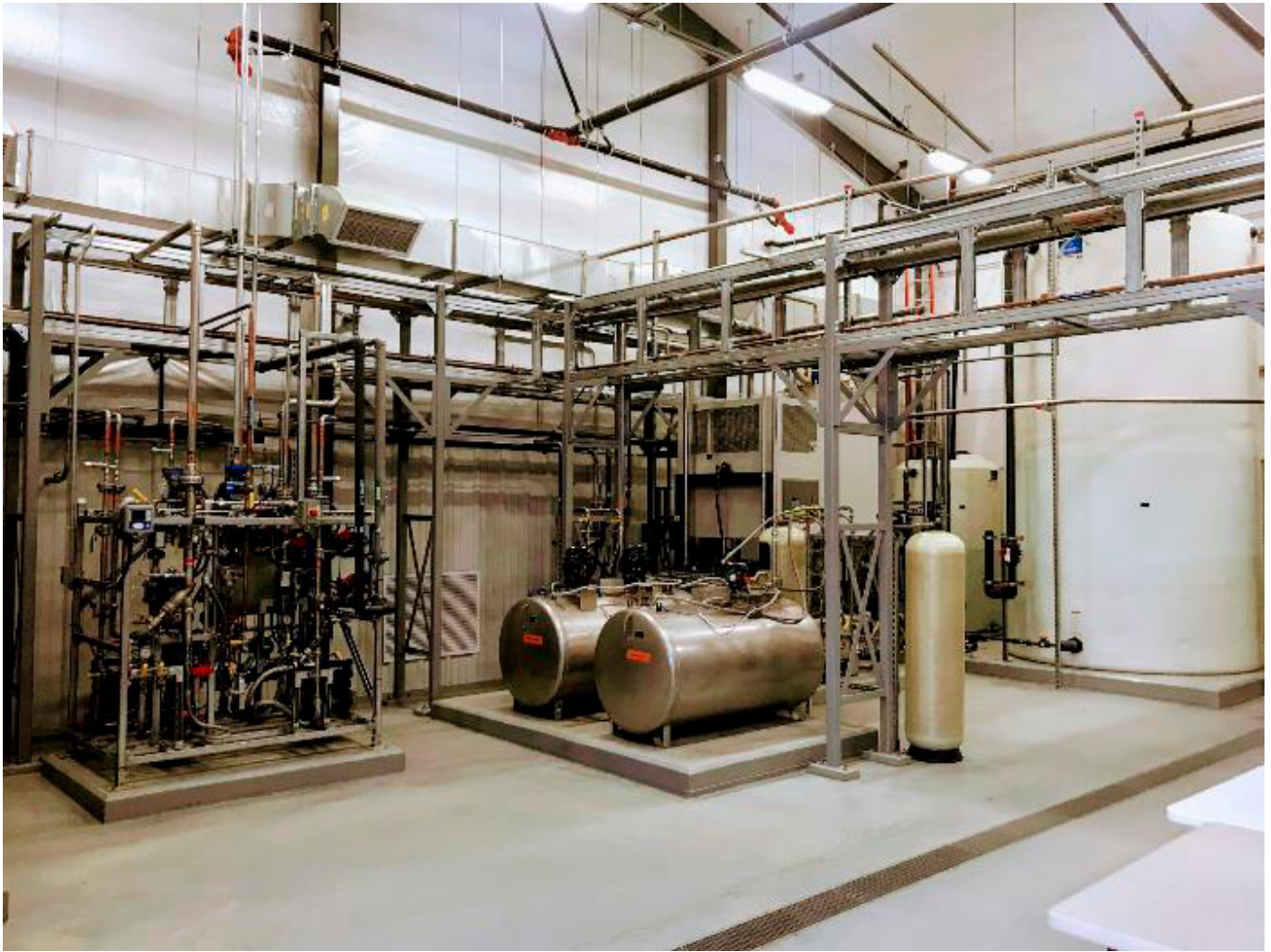
Figure 15-14. Resin regeneration system.
