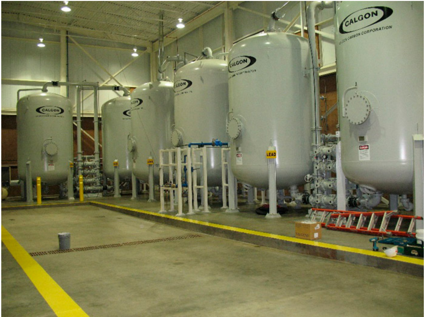
Figure 15-6. GAC treatment system, Oakdale, MN. Source: Courtesy of the Minnesota Department of Health.
