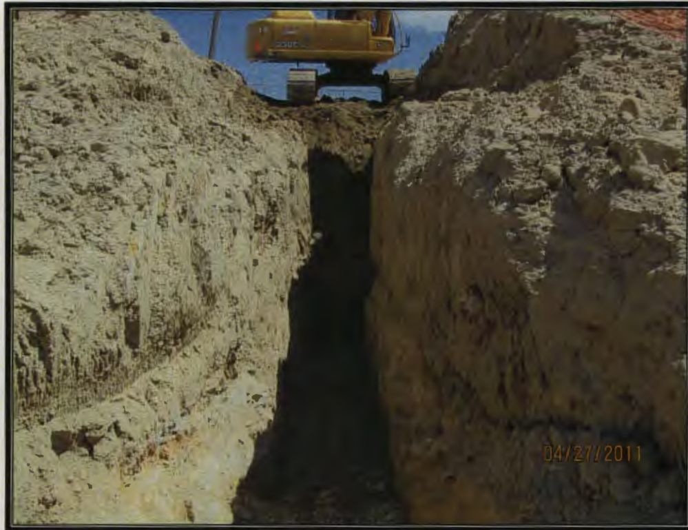
Photo 3: Removing the Leak Detection System
