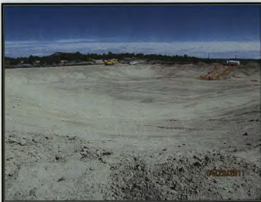
Photo 6: Pond after Liner and Leak Detection Removed
