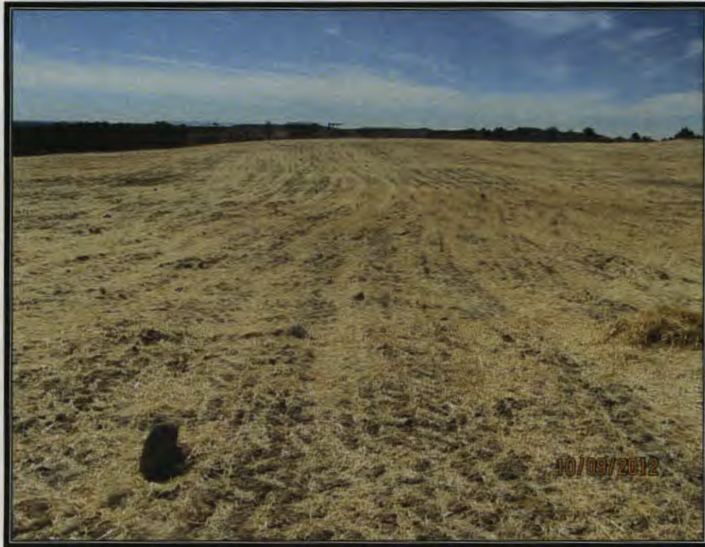
Photo 8: Pond after Backfill and Reclamation (View 3)
