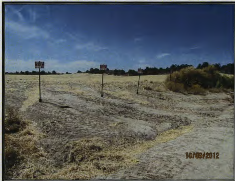
Photo 7: Pond after Backfill and Reclamation (View 1)
