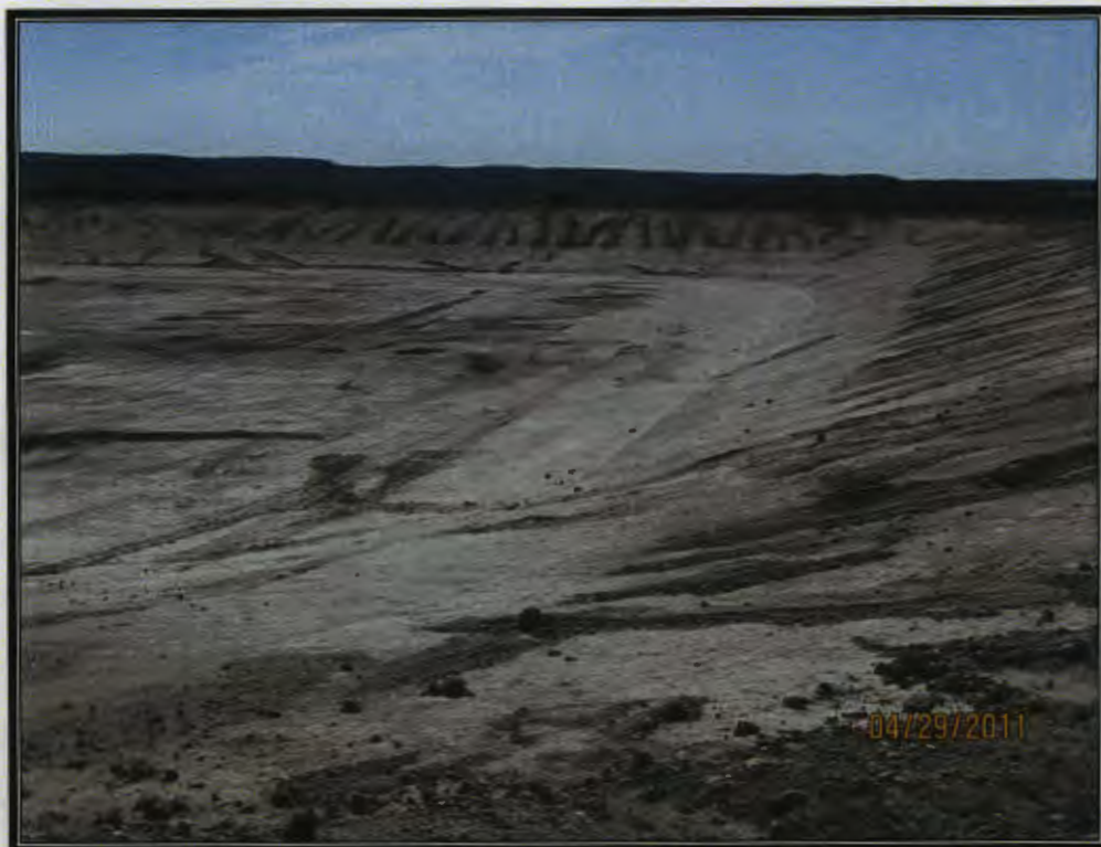
Photo 5: Pond after Liner Removal
