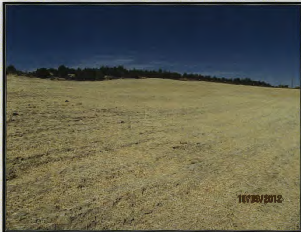
Photo 8: Pond after Backfill and Reclamation (View 4)
