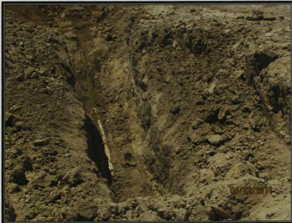
Photo 2: Removing the Leak Detection System
