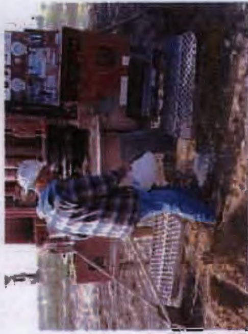
Plugging soil bore
