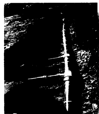
New Sparging Tubes were added to the system
