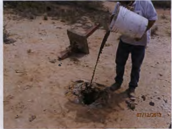
Plugging MW-1 with a 1-3% bentonite/concrete slurry with a 3 ft concrete cap, facing south 7/12/12
