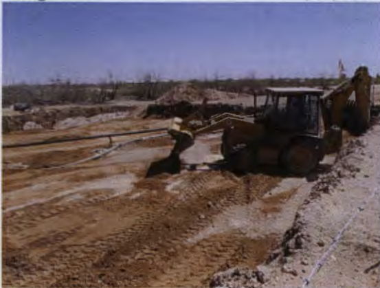
Installing 6" bottom sand pad, facing northeast 4/29/2013
