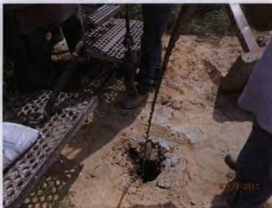
Plugging MW-2 with a 1-3% bentonite/concrete slurry with a 3 ft concrete cap, facing south 7/12/12
