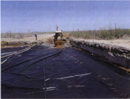
Installing a 1' sand pad above liner, facing east 4/29/2013
