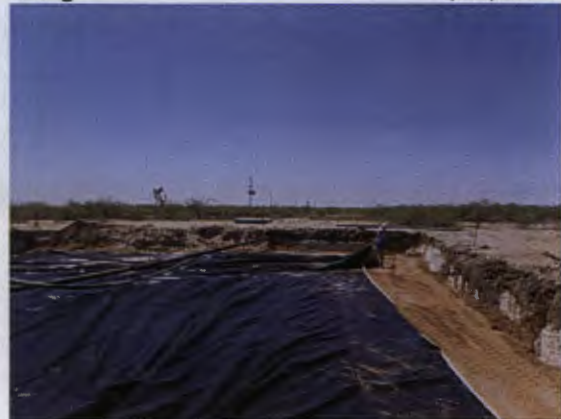
Installing 76'x77', 20-mil reinforced plastic liner at 5' bgs, facing west 4/29/2013
