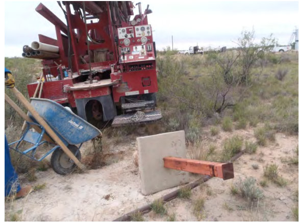
Plugging MW-3 with a 1-3% bentonite/concrete slurry and a 3 ft concrete cap, facing SE 10/25/13
