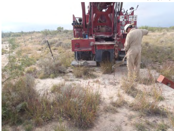
Plugging MW-4 with a 1-3% bentonite/concrete slurry and a 3 ft concrete cap, facing south 10/25/13
