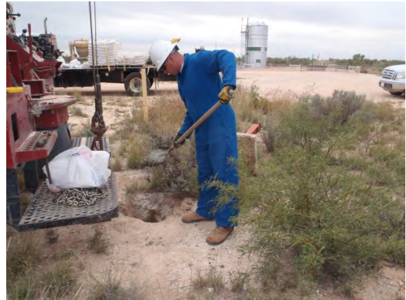
Plugging MW-1 with a 1-3% bentonite/concrete slurry and a 3 ft concrete cap, facing south 10/25/13
