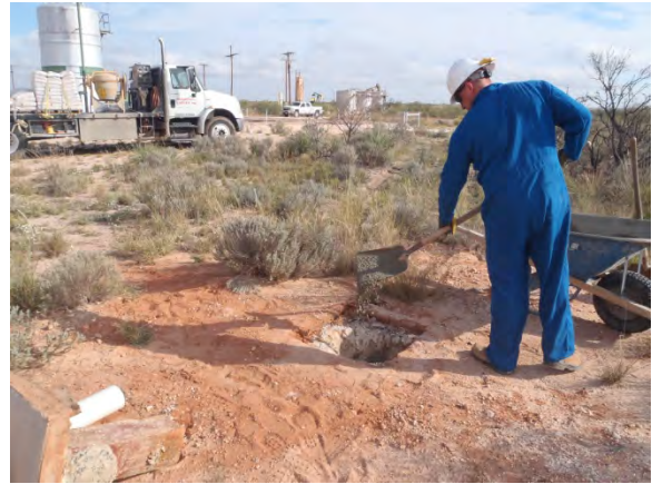
Plugging RW-1 with a 1-3% bentonite/concrete slurry and a 3 ft concrete cap, facing northwest 10/25/13
