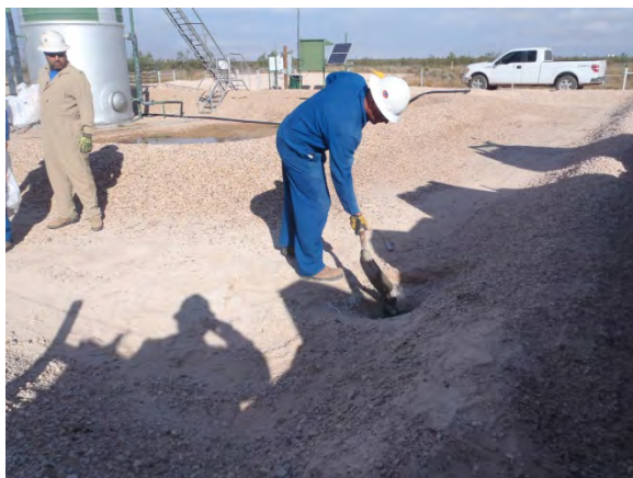
Plugging MW-2 with a 1-3% bentonite/concrete slurry and a 3 ft concrete cap, facing NW 10/25/13
