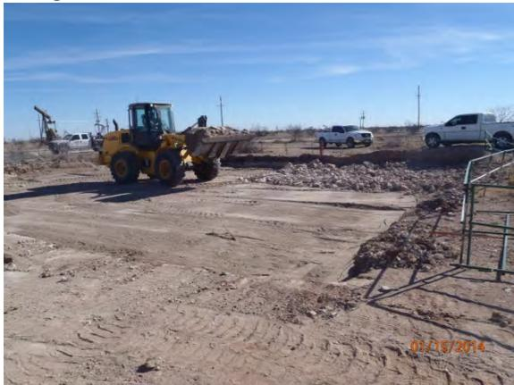
Backfilling the excavation with screened rock,
