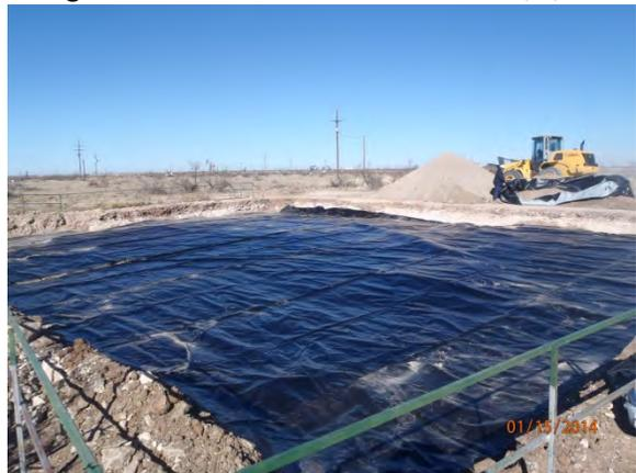
20-mil, reinforced liner installed,
