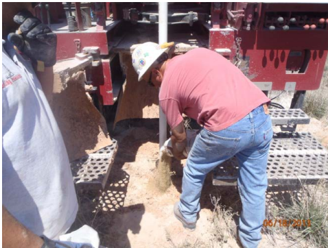
Installing the sand pack 6/18/13
