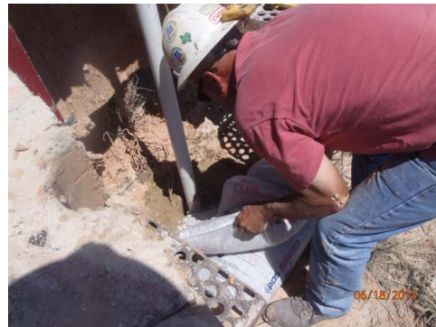
Installing the bentonite seal 6/18/13
