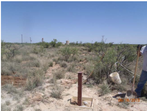
Installing the monitor well casing prior to cementing the monitor well in, facing north 6/18/13
