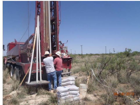
Installing the casing, facing northwest 6/18/13
