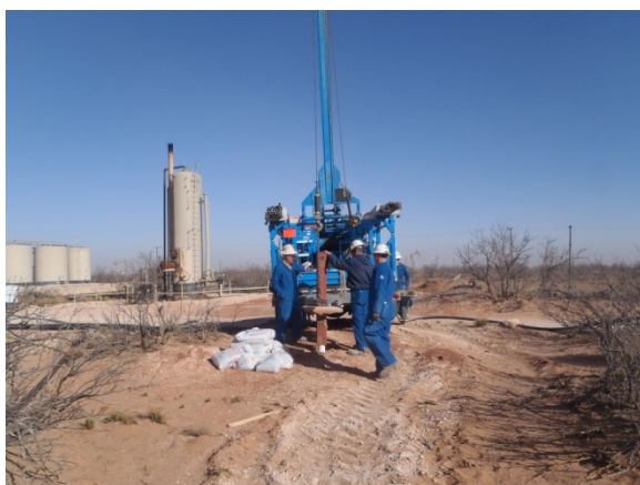
Removing MW-2, facing north 03/05/14
