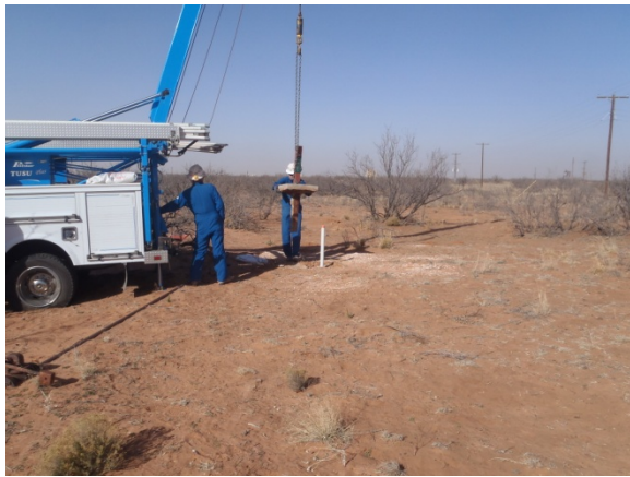
Removing MW-1, facing west 03/05/14
