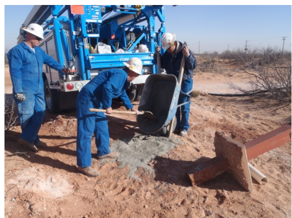
Plugging MW-2 with a 1-3% Bentonite/concrete slurry with a 3ft concrete cap, facing northwest 03/05/14
