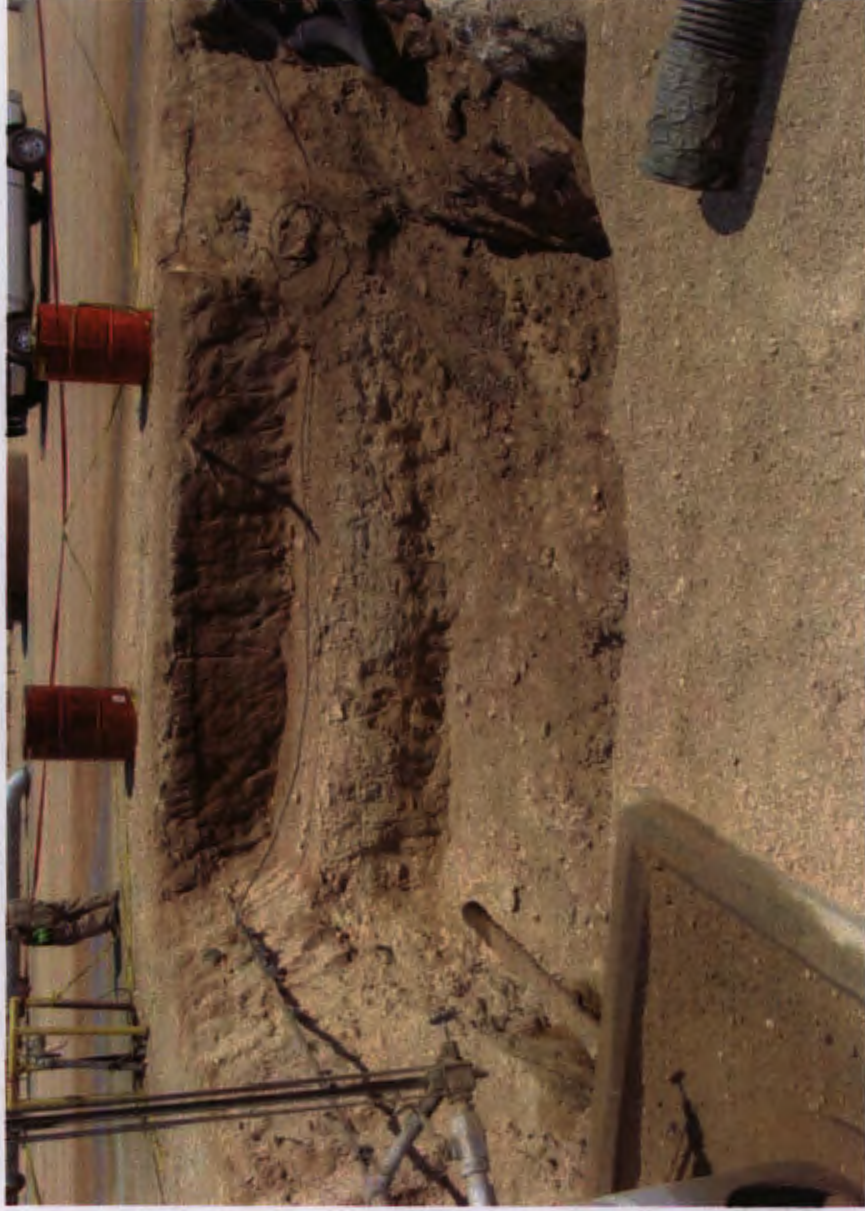
Figure 3: Final Excavation Extents, July 11, 2011 (Dimensions of the excavation are: 20' wide x 21' length and 13 ' in depth )
