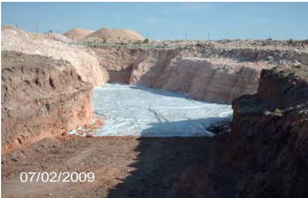
EK Queen Pearce 6-Inch - Liner Installation
