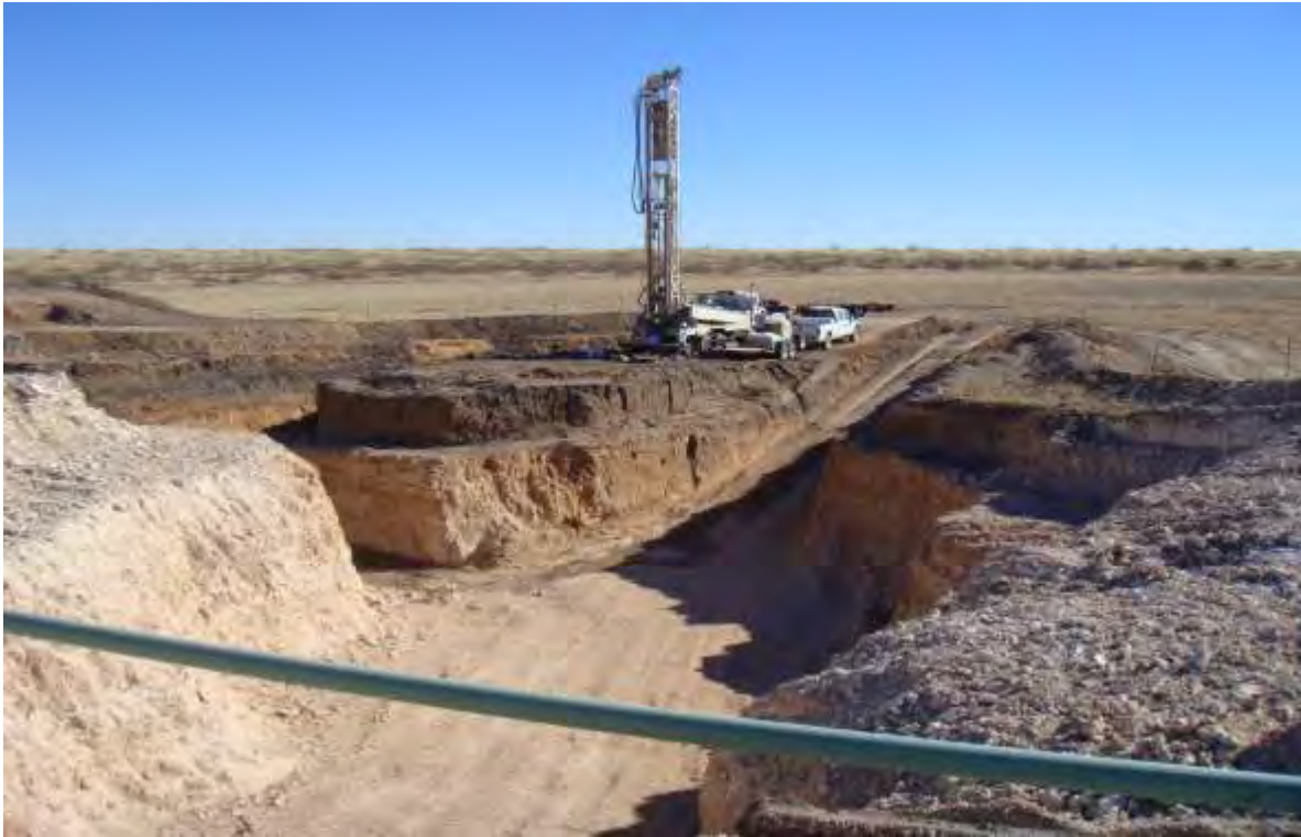
EK Queen Pearce 6-Inch – Installation of Monitor Well MW-3
