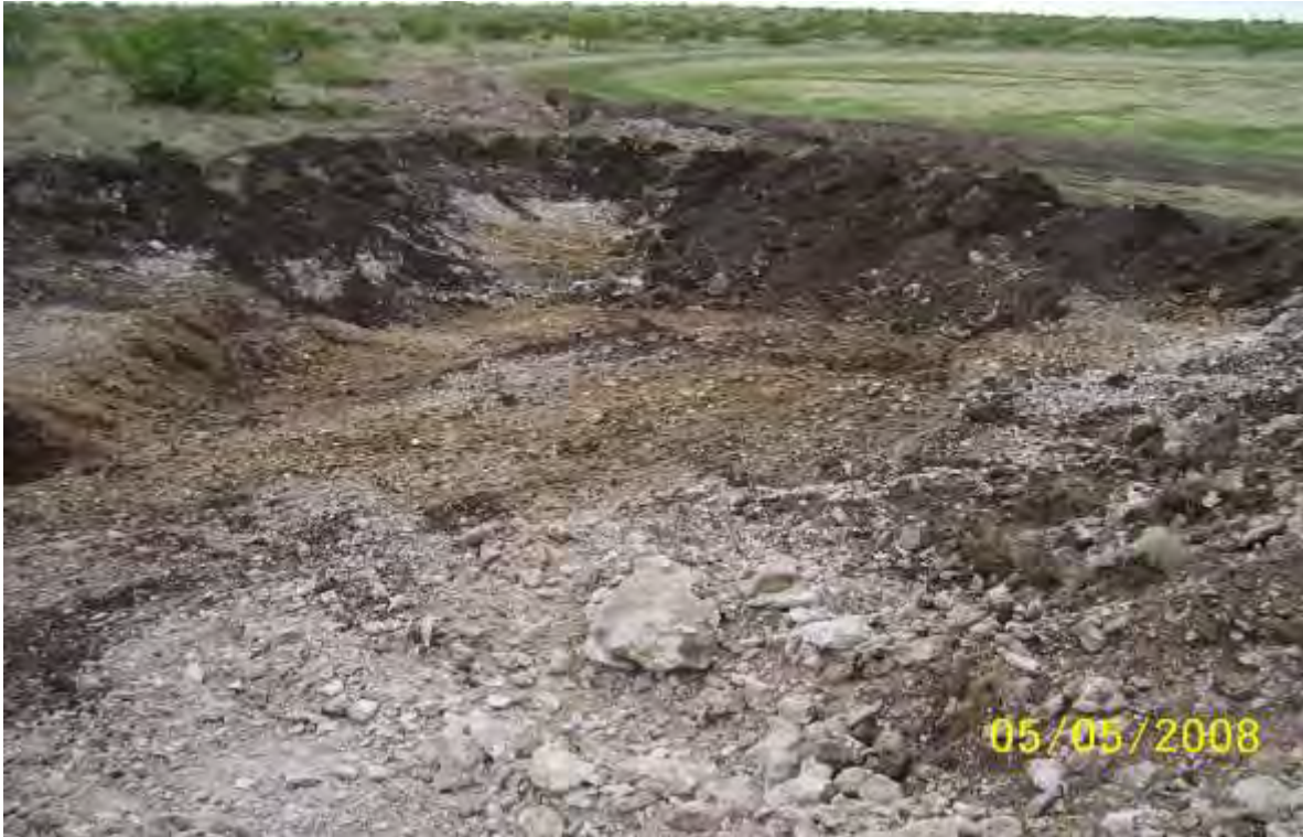
EK Queen Pearce 6-Inch – Excavation (Looking Southeast)
