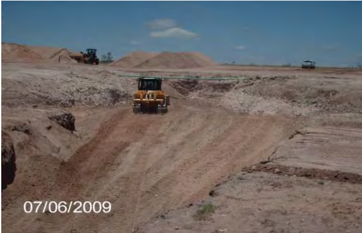
EK Queen Pearce 6-Inch - Backfilling
