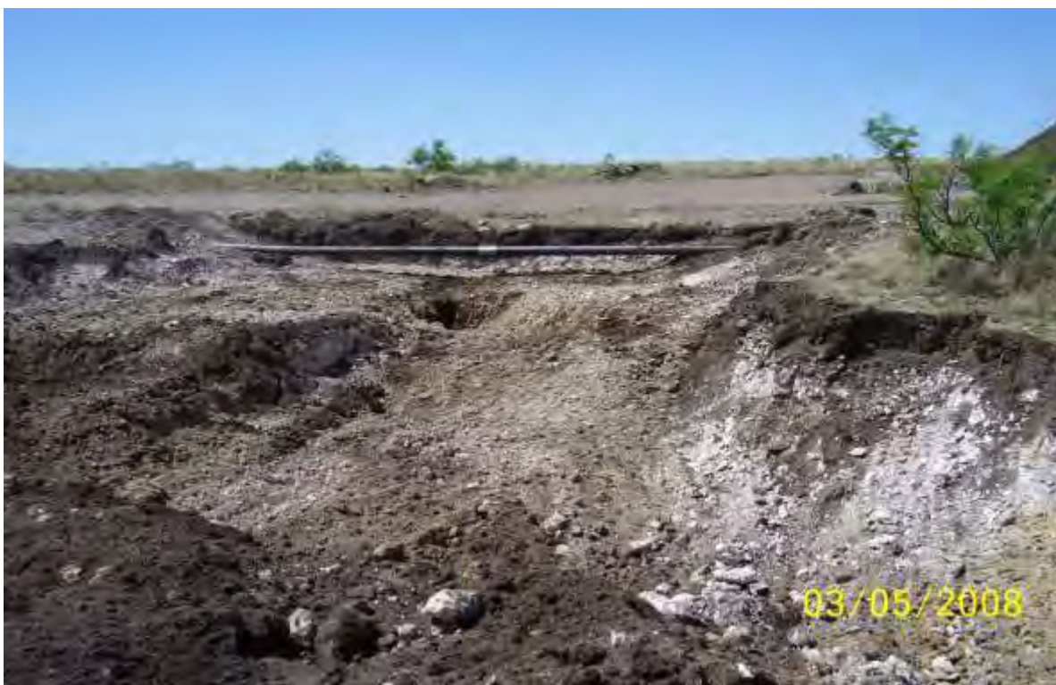
EK Queen Pearce 6-Inch – Excavation (Looking North)
