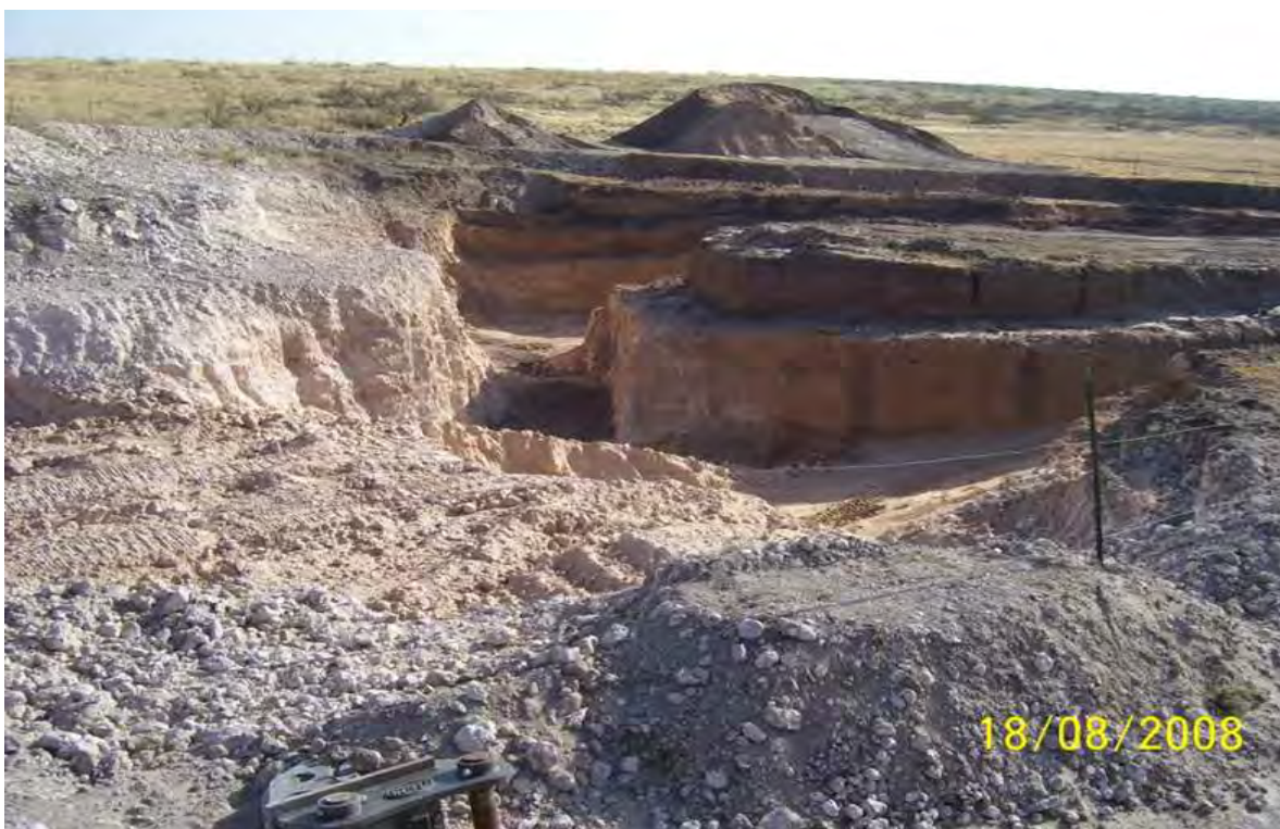
EK Queen Pearce 6-Inch – Excavation (Looking East)
