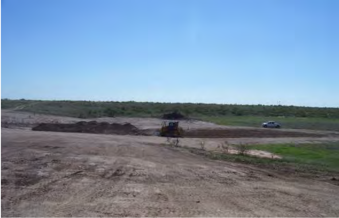
EK Queen Pearce 6-Inch – Backfilling (Near Completion, Looking East)
