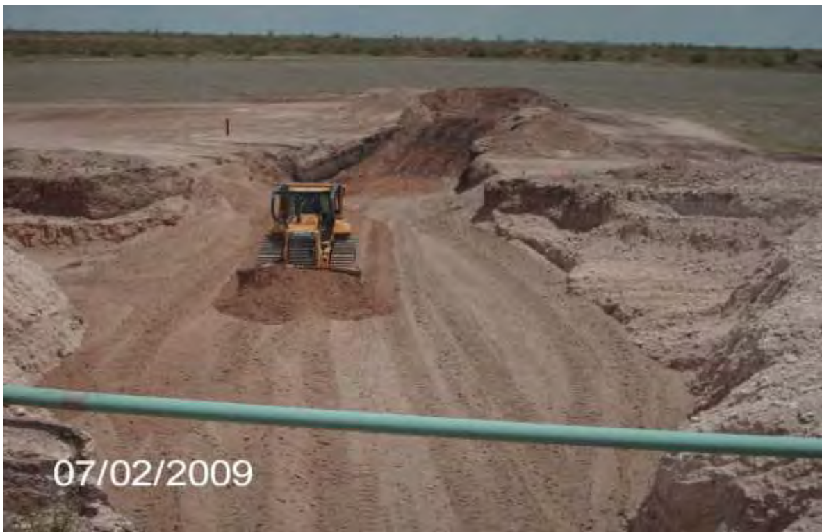
EK Queen Pearce 6-Inch - Backfilling
