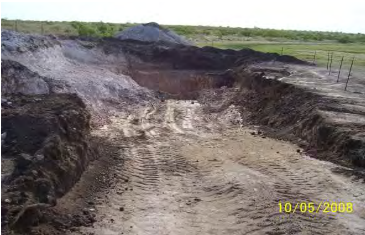
EK Queen Pearce 6-Inch – Excavation (Looking Southeast)
