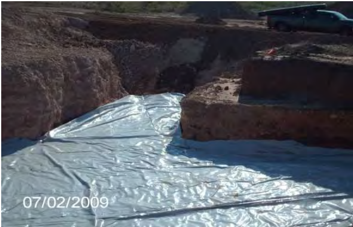
EK Queen Pearce 6-Inch - Liner Installation
