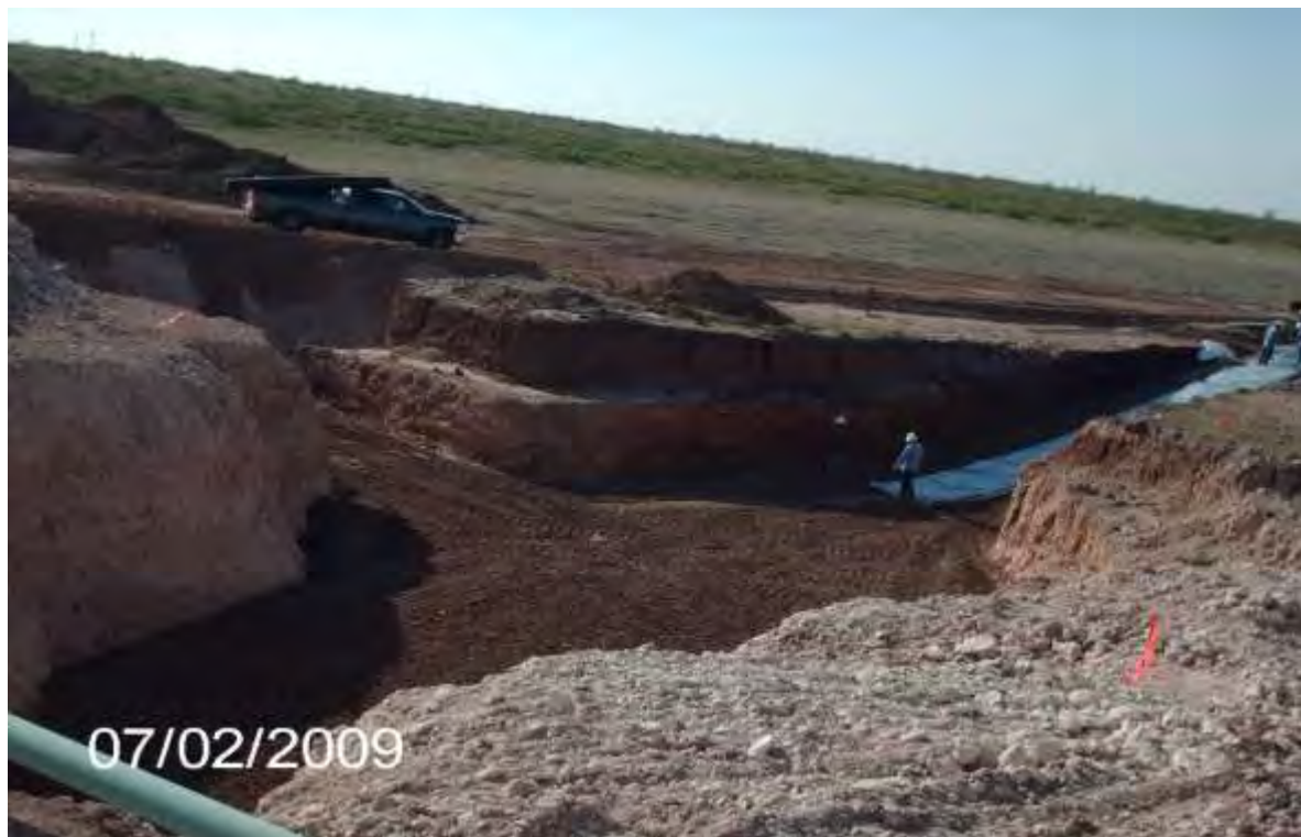
EK Queen Pearce 6-Inch – Liner Installation
