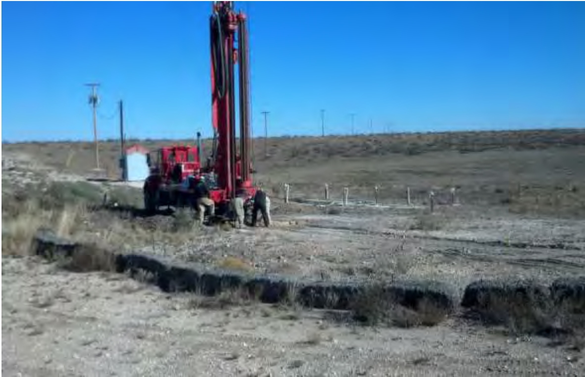
EK Queen Pearce 6-Inch – Installation of Monitor Well MW-4
