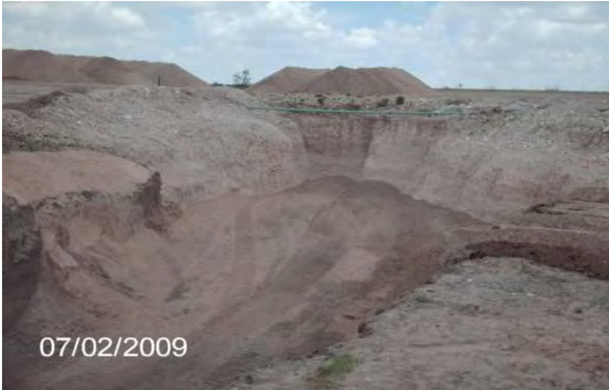
EK Queen Pearce 6-Inch - Backfilling
