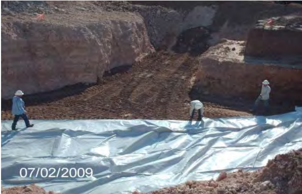
EK Queen Pearce 6-Inch - Liner Installation
