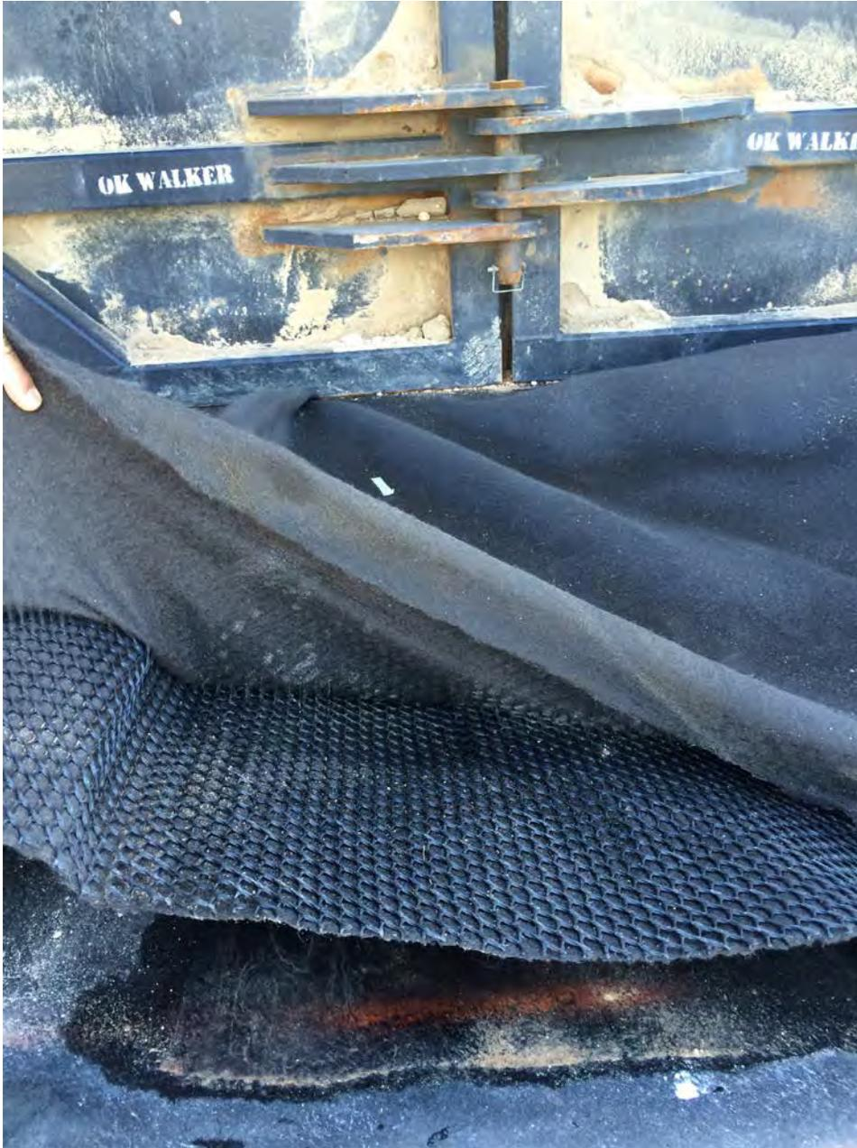
Photograph of 40-mil secondary liner (bottom), 200-mil geogrid drainage system with attached geotextile beneath and over the grid. This leak detection system extends about 4-feet beyond the walls of the AST.
