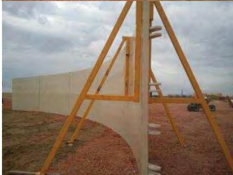
As the panels are moved from the truck to the site, personnel should be ready with ladders, dead blow hammers and pins to assemble and secure the panel connecting plates. The telehandler will position the panel to allow the connecting plates on the end of the panel to align the adjoining panels connecting plate such that the thru holes are centered on one another. 6 pins should be used to join panels at connecting points. The picture below shows pins with latch pins secured.
