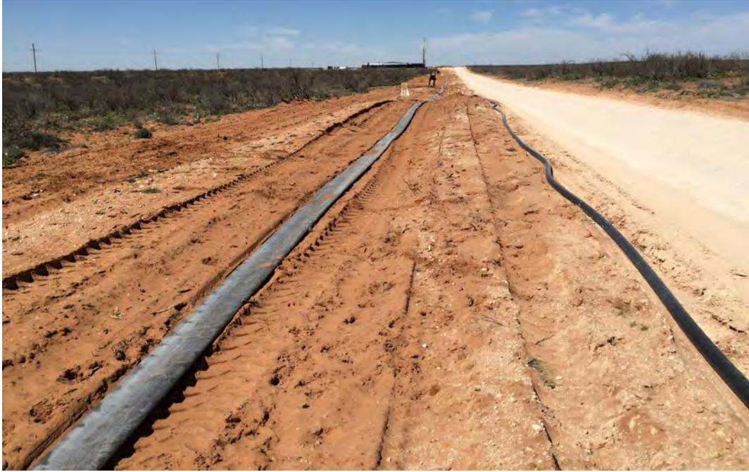
Lay flat hoses to transport produced water between ASTs. These same style of hoses will be used to transport produced water to hydraulic stimulation of individual wells.
