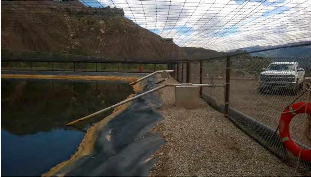
*Figure B-1: The secondary fence system supports the netting and excludes wildlife. Rather than chain link fencing as shown above, McElvain will employ 4-strand barbed wire. The pipes leading from the containment to the work area outside of the fence are for pumping water to E&P activities. The small pipe between the steel pipes is the riser for the leak detection system.*
