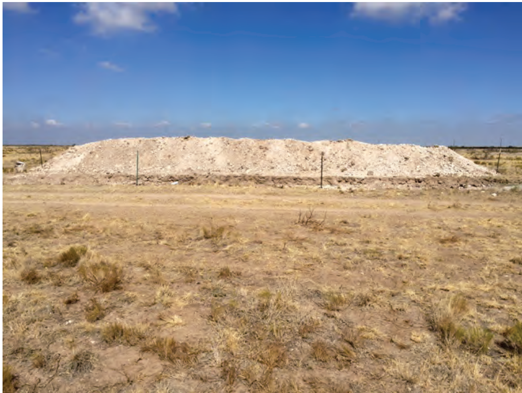
Photo 5 – View to west at soil stockpile on west side of repair excavation.
