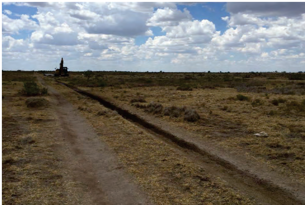
Photo 2 – View to south at hydrotest water spill path along west side of patrol road on July 25, 2016.
