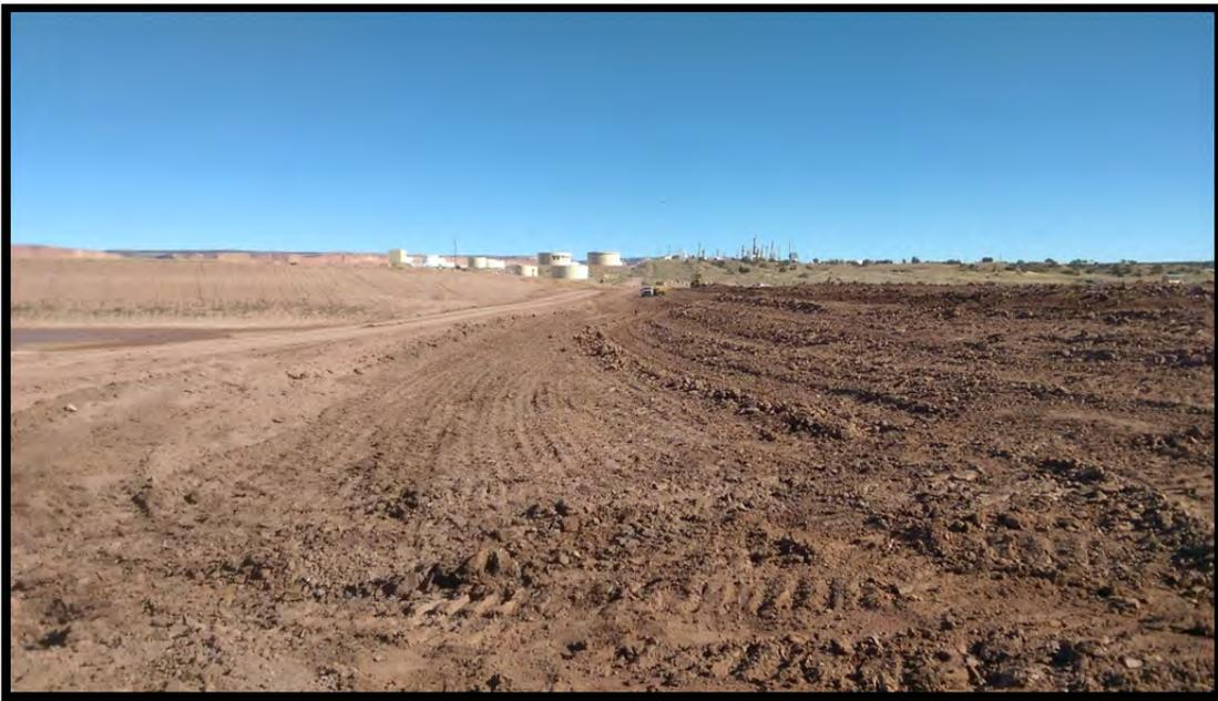
**Photo #22:** Pond 9 North Berm Completed.
