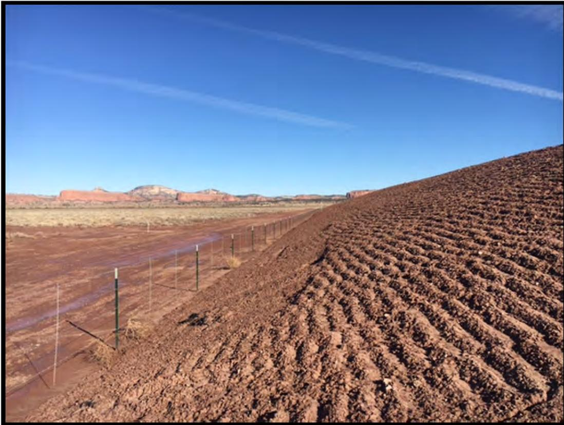
**Photo #14:** Pond 7/8 West Berm Completed Fill.
