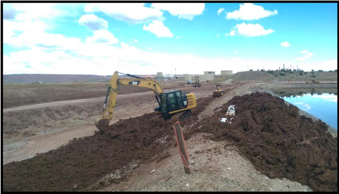
**Photo #21:** Pond 9 Start of Fill Placement on North Berm
