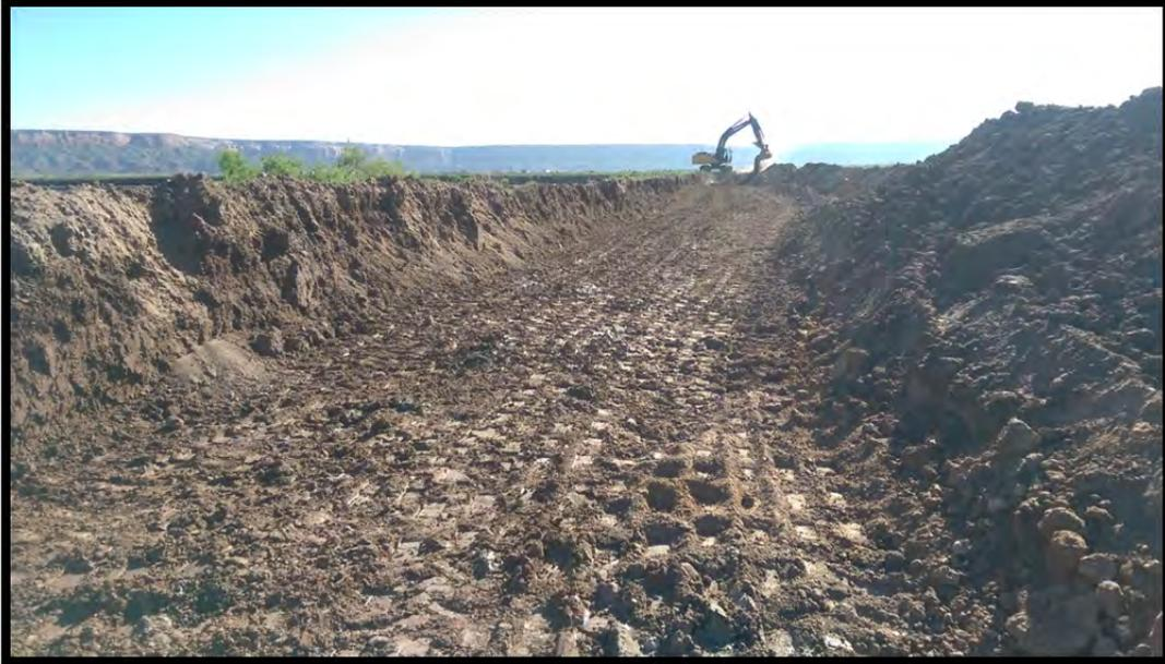
**Photo #17:** Pond 11-12 Berm Being Removed and Reworked
