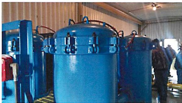
20micron/5micron Filtration Unit
