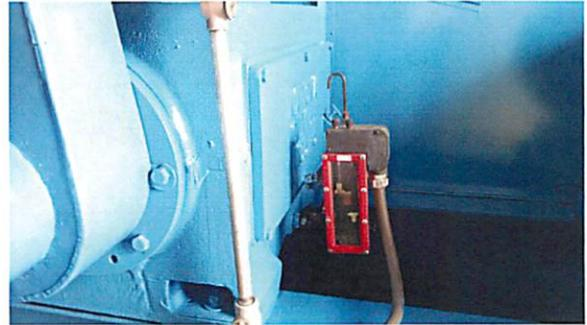
Pump lubrication fluid level meter
