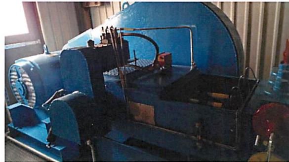
Pump No. 2 in Pump House (two large pumps capable of ~ 155 gpm)
