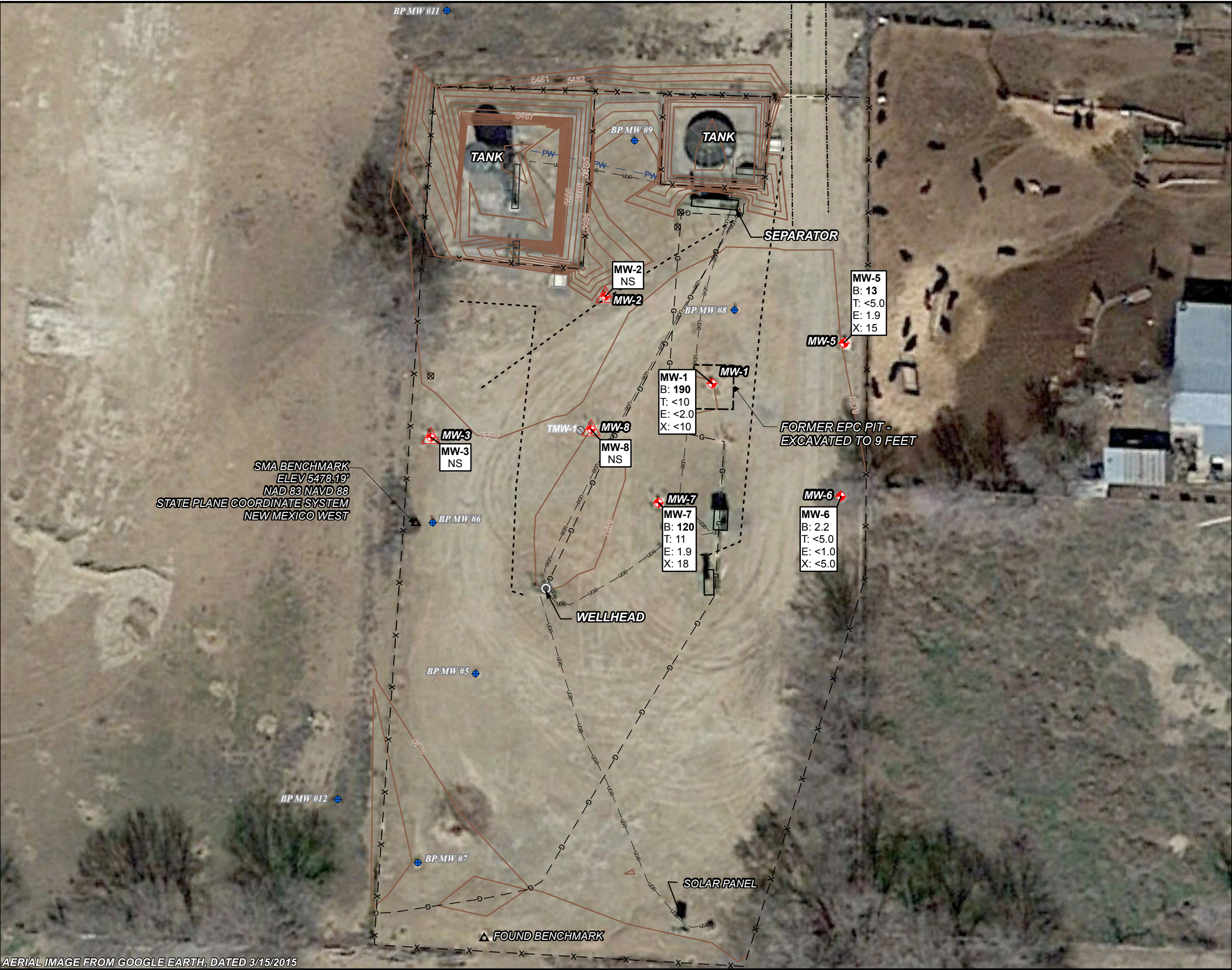
AERIAL IMAGE FROM GOOGLE EARTH, DATED 3/15/2015
