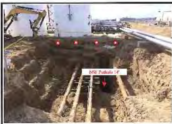
Photo # 5 West Wall Composite Sample & NW Pothole 14'
