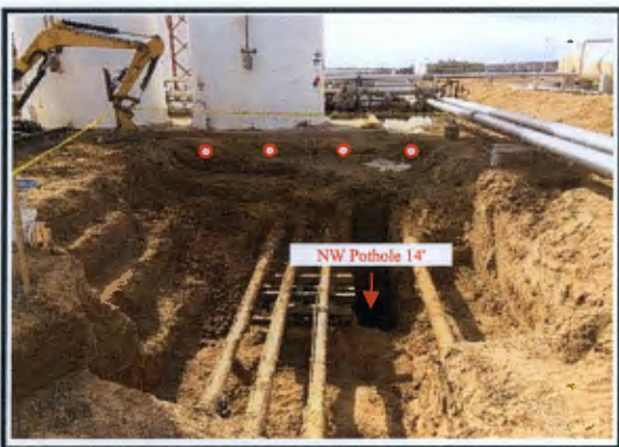
Photo # 5 West Wall Composite Sample & NW Pothole 14'
