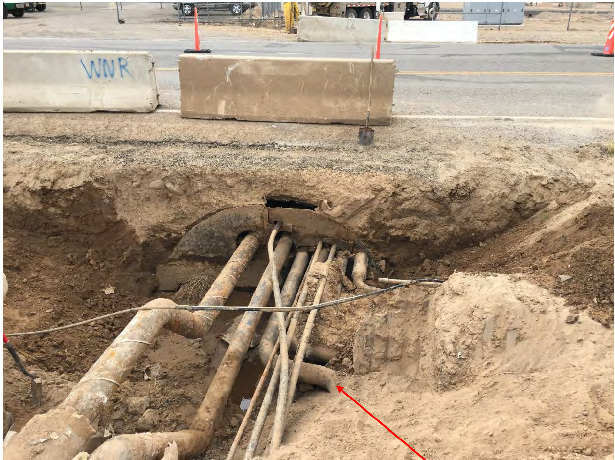
Picture of excavation looking south at County Road 4990.
