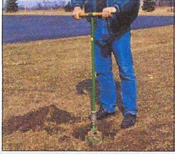
A 12 inch (300 mm) hole is augered to a depth of about 3 1/2 feet (1050 mm).
