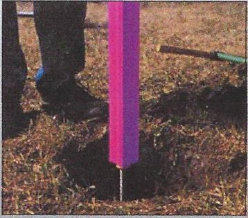
The finned sleeve (filled with grease) is placed over the rod and the datum point added (or filed onto the rod end).
