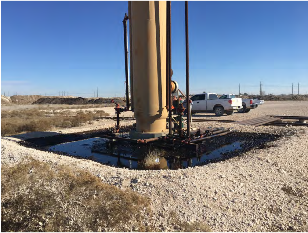
Release (Looking Northeast)
