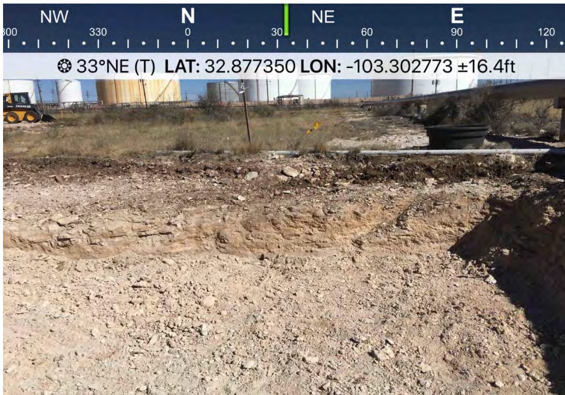
Photo 4. Northeast side of excavation. January 24, 2019.
