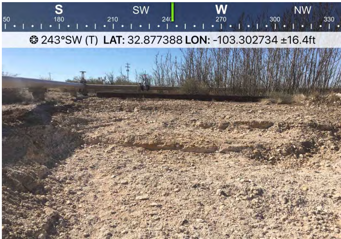
Photo 2. Southwest/south sides of excavation. January 24, 2019.
