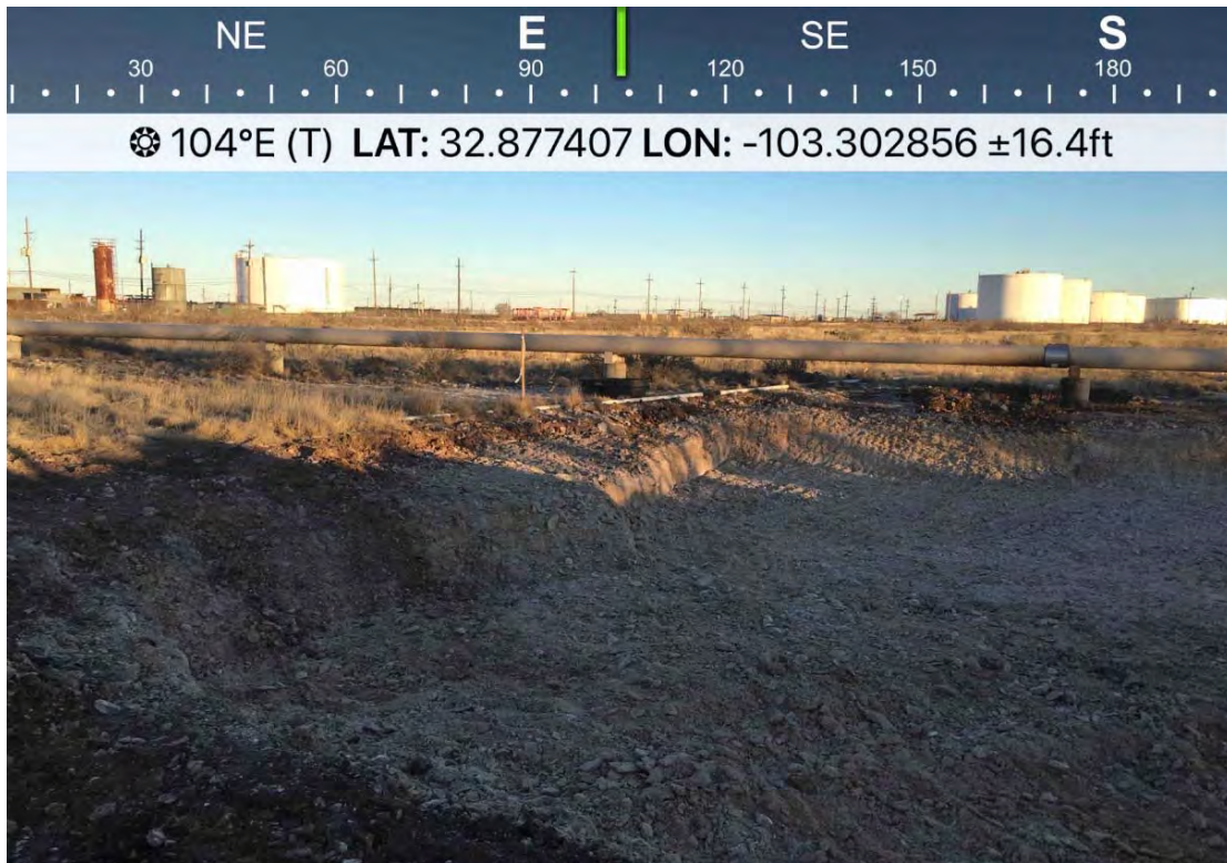
Photo3. Northeast/east side of excavation. January 23, 2019.
