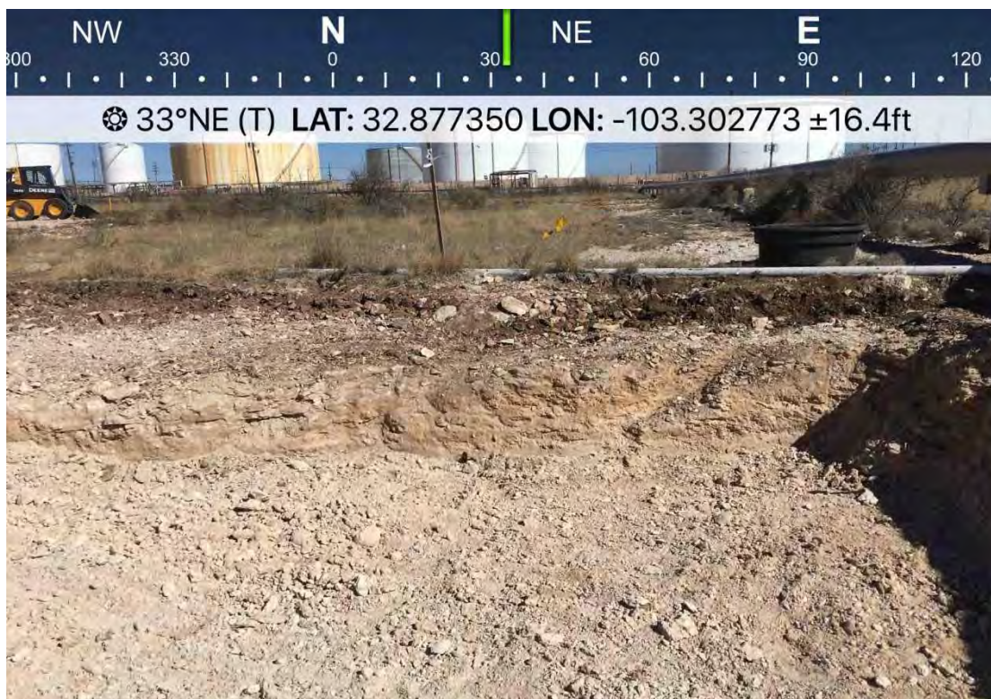
Photo 4. Northeast side of excavation. January 24, 2019.
