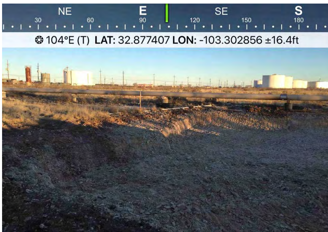
Photo3. Northeast/east side of excavation. January 23, 2019.
