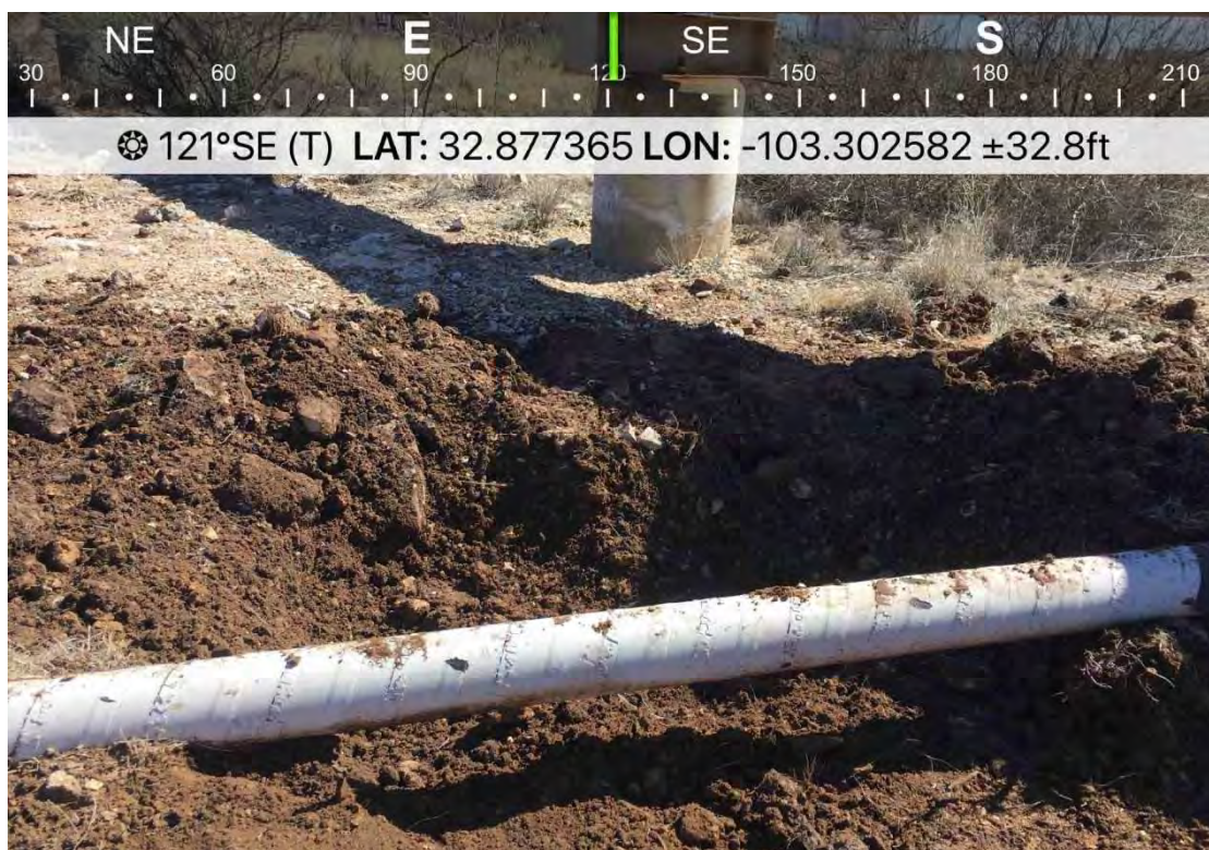
Photo 5: Additional soil removal along northeast/east corner of excavation (ES-01-R2). March 15, 2019.
