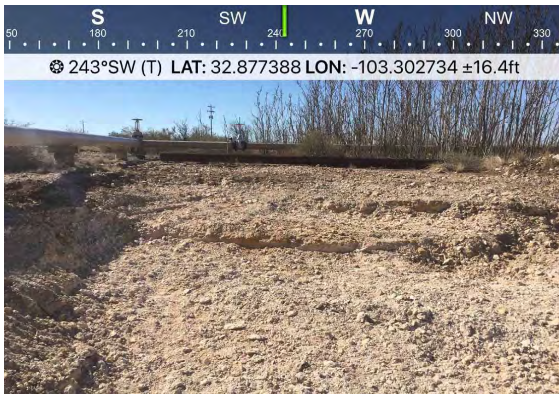
Photo 2. Southwest/south sides of excavation. January 24, 2019.
