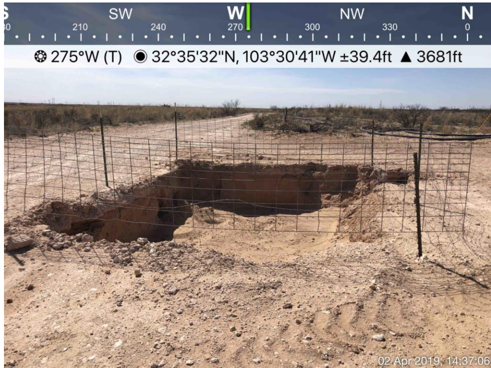
DP-3 Excavation Viewing West, April 2, 2019
