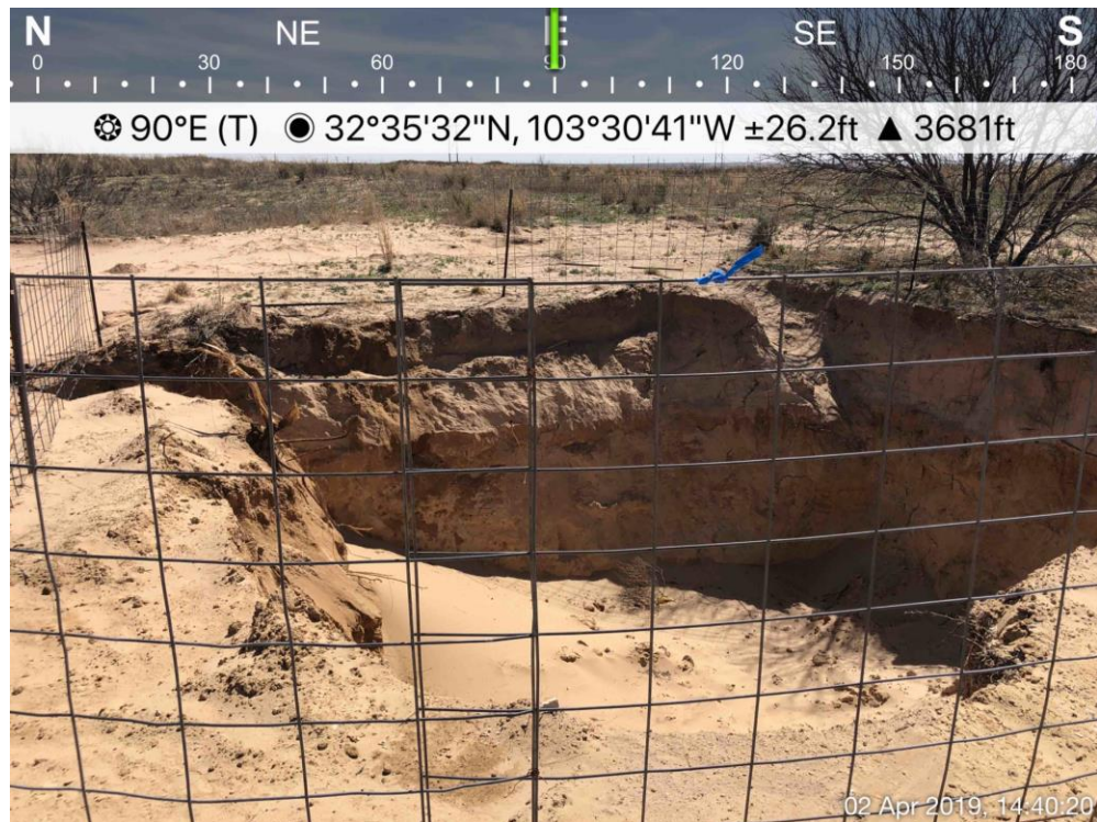
DP-8 Excavation Viewing East, April 2, 2019
