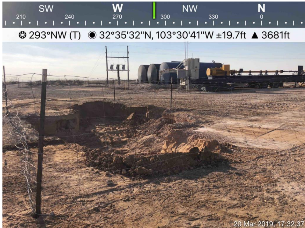
DP-9 Excavation Viewing Northwest, March 20, 2019
