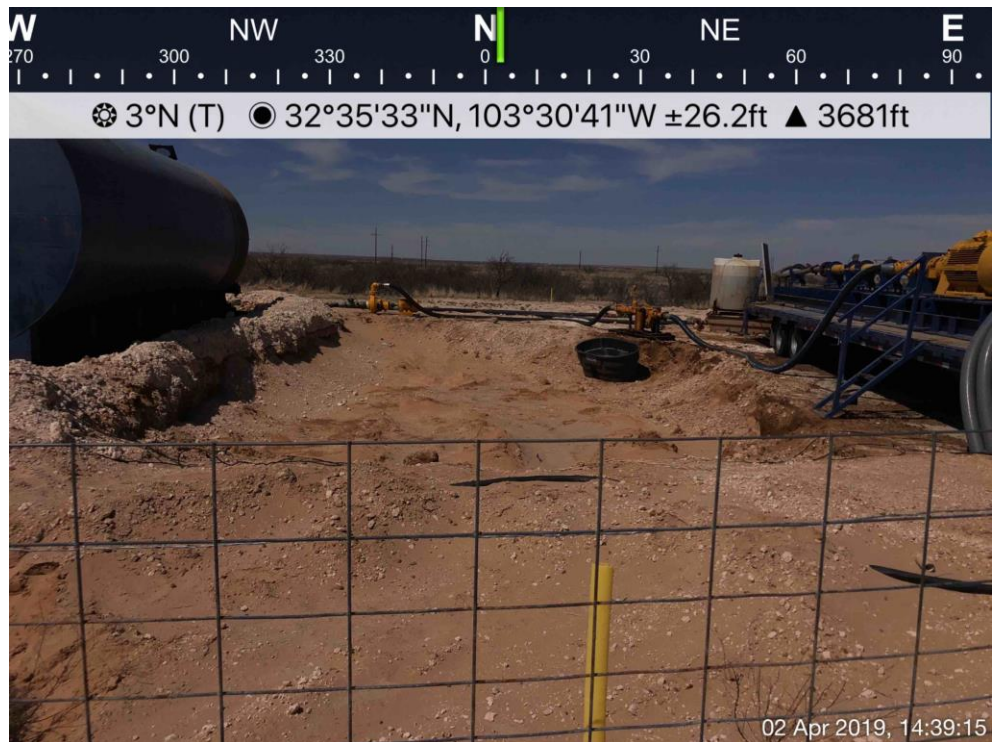
DP-6 and DP-7 Excavations Viewing North, April 2, 2019
