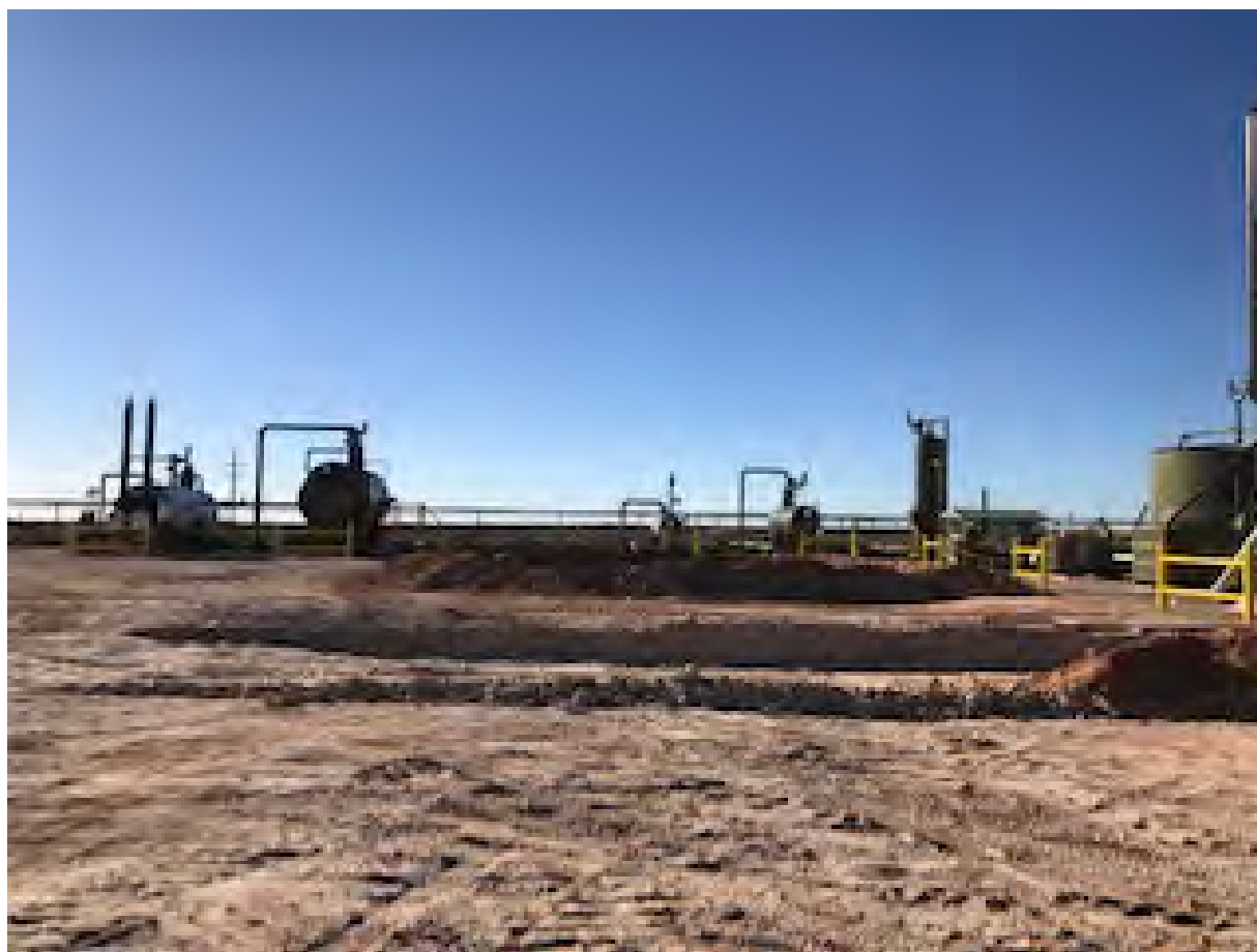
West facing view facing of the excavation.
