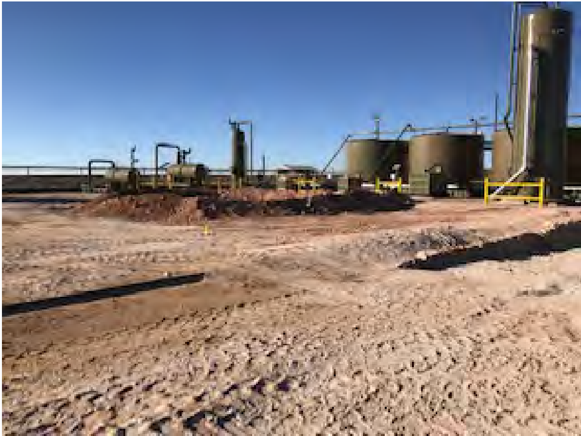
Northwest facing view of the excavation.
