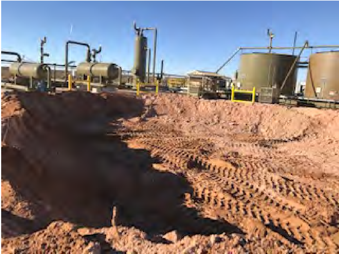
Northwest facing view facing of the excavation.
