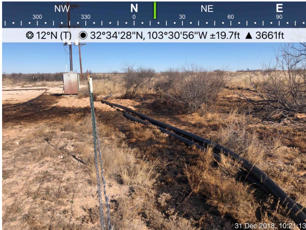
Spill Area Viewing North, December 31, 2018
