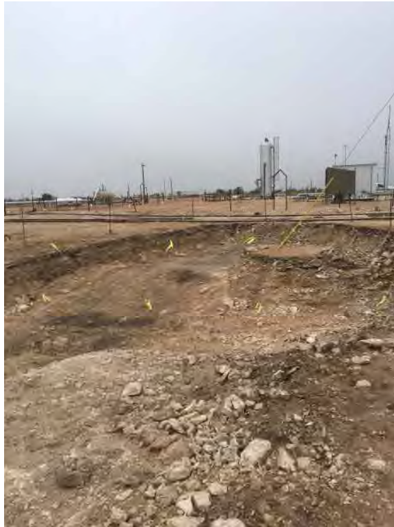
3.) View West - Central portion of excavation, Satellite Facility in background
