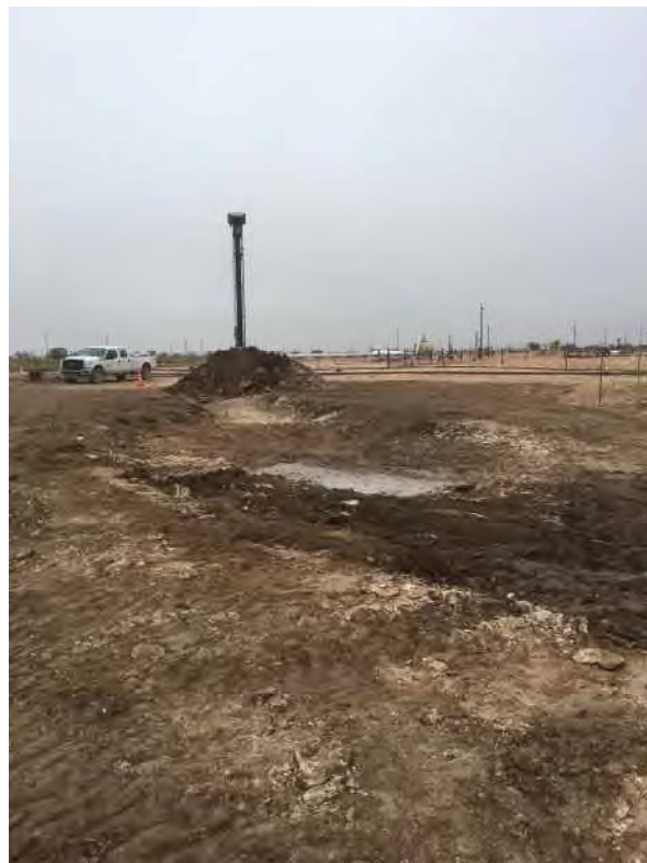
4.) View West - Central portion of excavation near AH-VERT2, Flare stack in background
