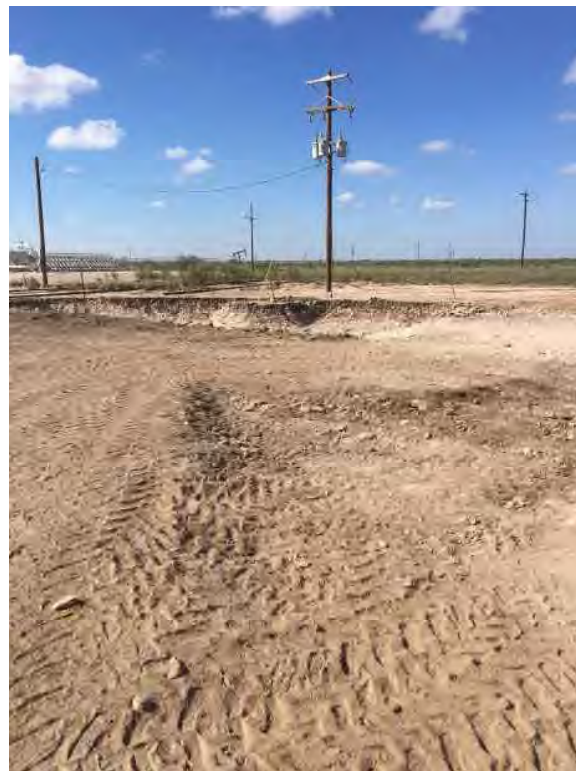
8.) View Northwest – Overview of completed excavation area in central portion.
