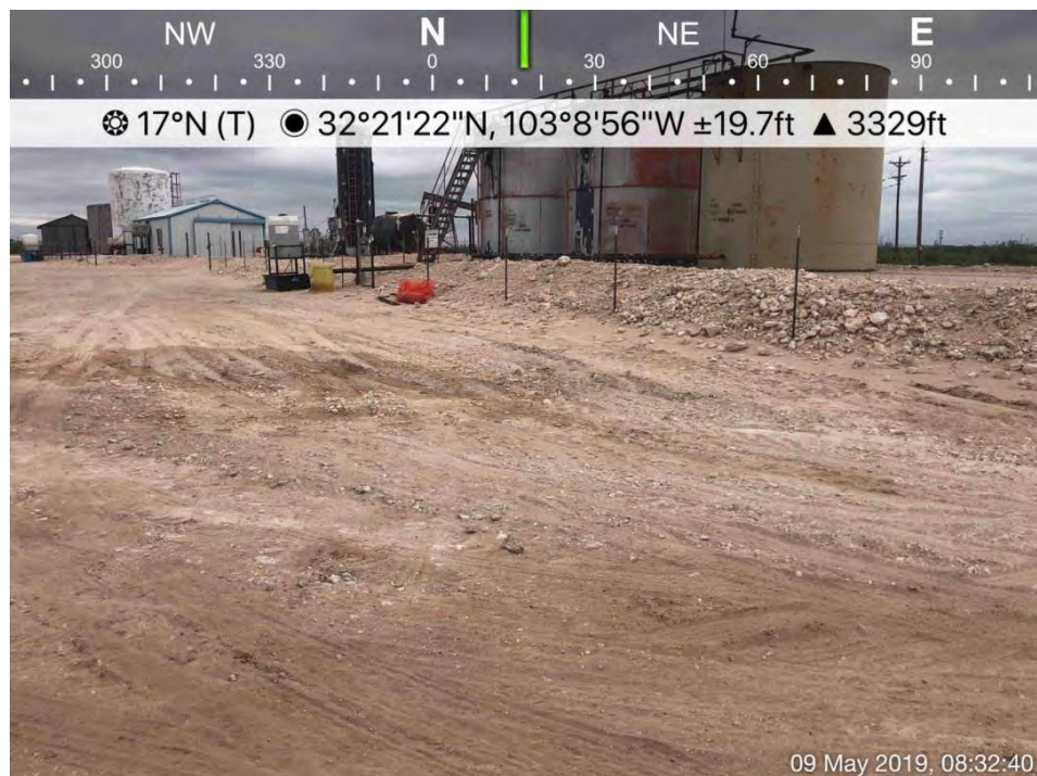
Backfilled Area near DP-20 viewing North, May 9, 2019
