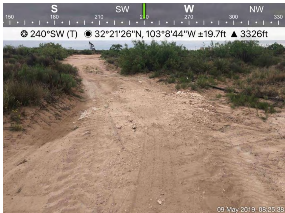
Backfilled Area near DP-11 Viewing West, May 9, 2019
