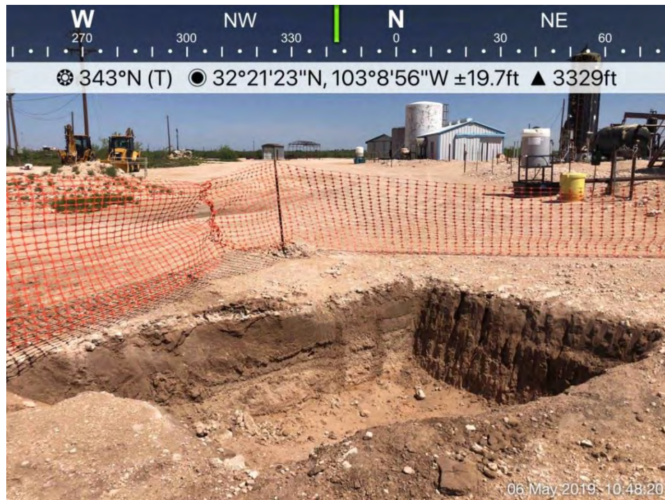
DP-20 Excavation viewing North, May 6, 2019
