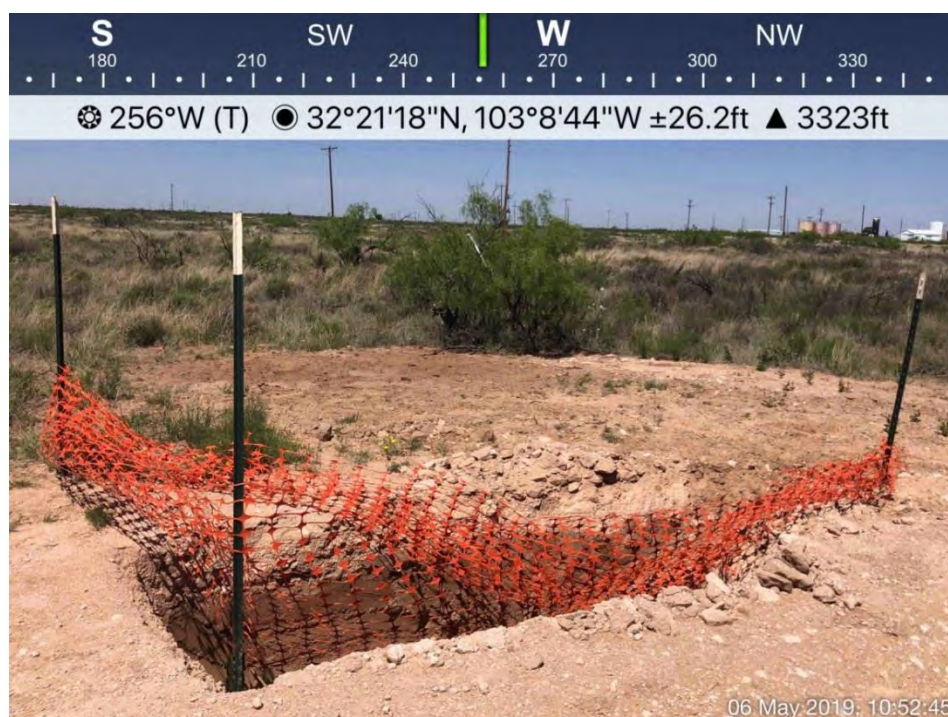
DP-3 Excavation Viewing West, May 6, 2019
