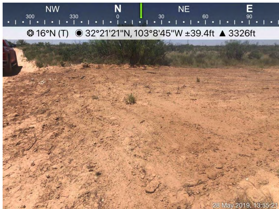
Backfilled and Seeded Area near DP-4 Viewing North, May 28, 2019
