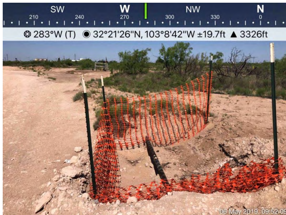
DP-9 Excavation Viewing West, May 6, 2019
