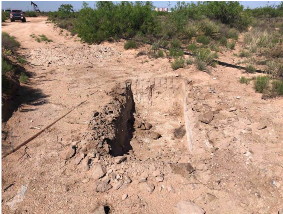
DP-11 Excavation viewing West, May 6, 2019
