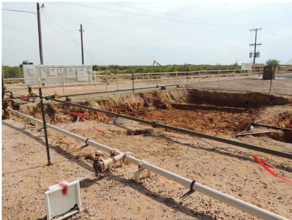
View Northwest– Area of AH-2
