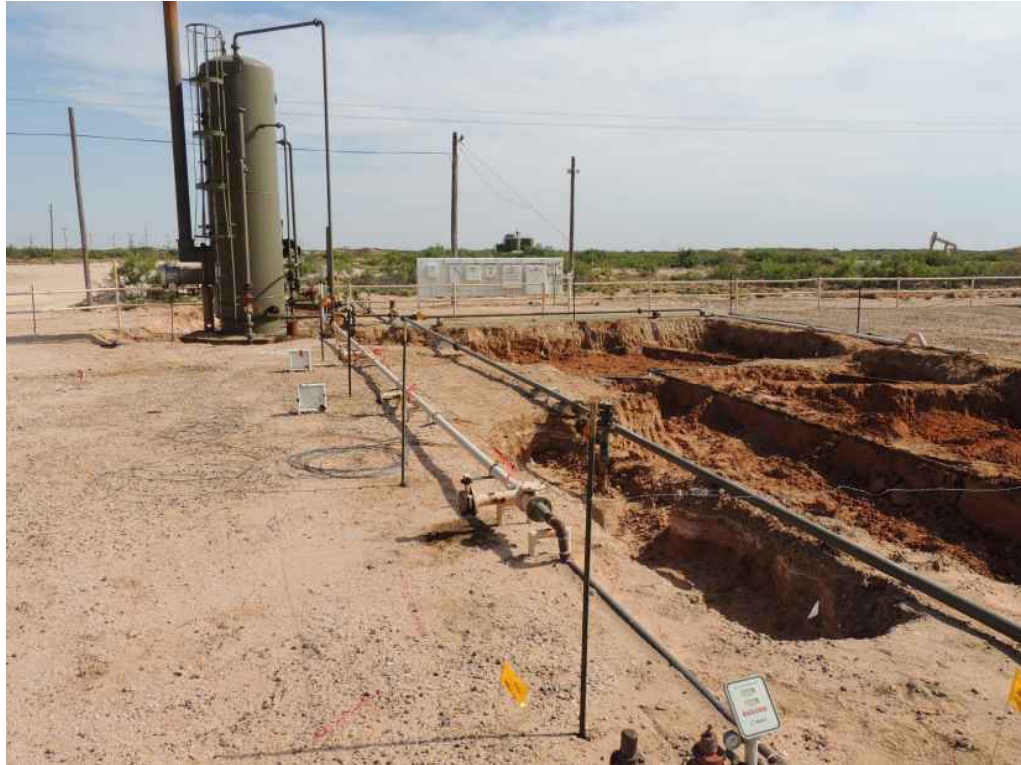
View Northwest – Area of AH-1 and AH-2
