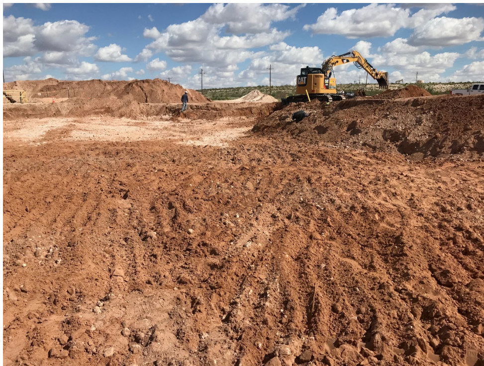
Photograph 1: View southeast of excavation.
