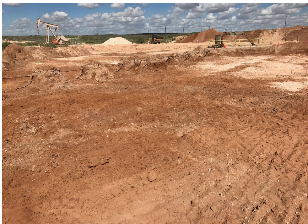
Photograph 2: View northeast of excavation.
