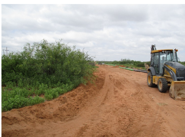
5. View of OWL pipeline right-of-way, facing west.
