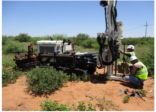
2. View of advancement of SB-03, facing north.
