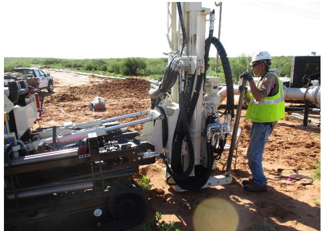
4. View of advancement of SB-12 near release point, facing northwest.
