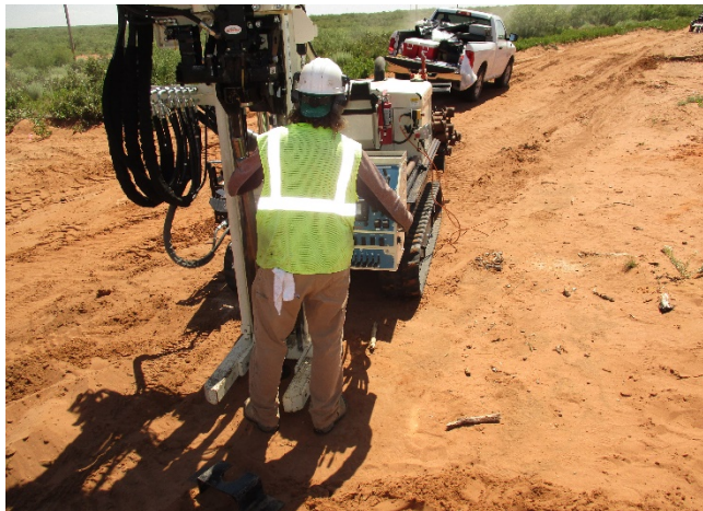
3. View of advancement of SB-08 in pipeline right-of-way, facing northeast.
