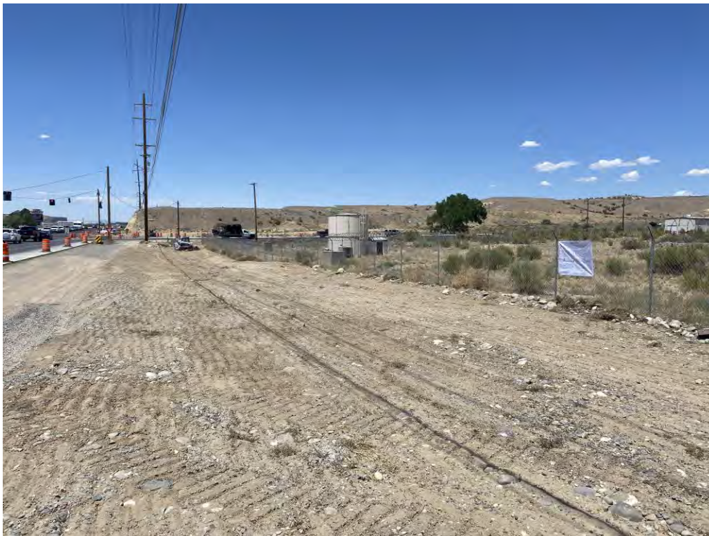
Photograph 4: View of sign from HWY 64 looking West towards the intersection with CR 350
