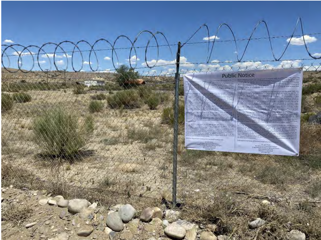
Photograph 3: View of sign from HWY 64 looking Northwest towards the infiltration gallery.
