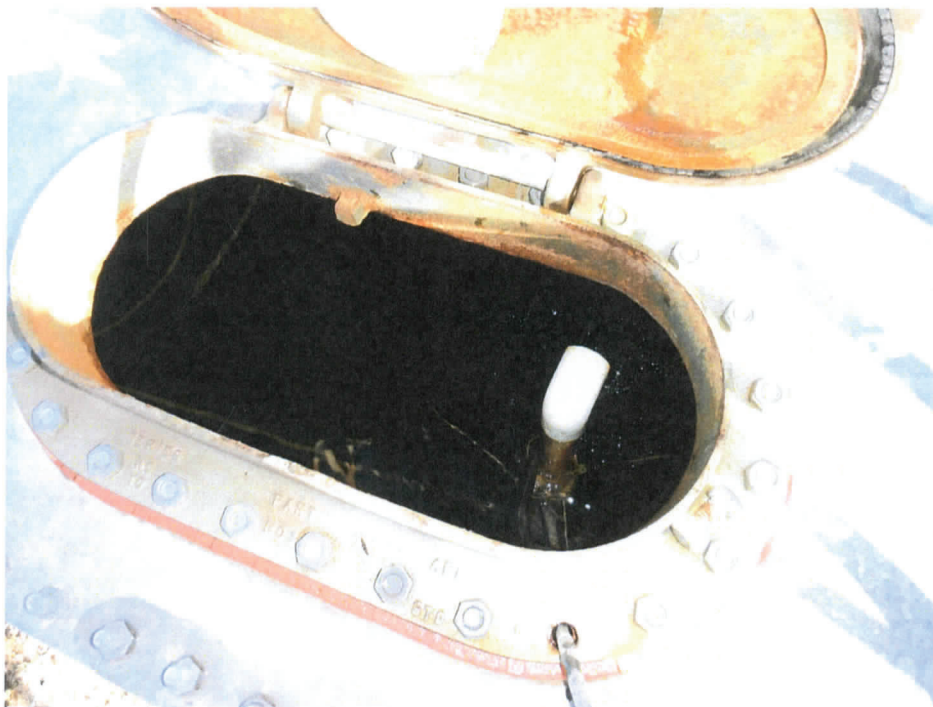
Photo 10 - Discharge point inside collection tank for ICP-DHR-10 ("James East Well").
