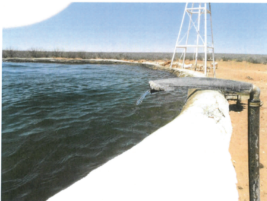
Photo 6 - Discharge point for ICP-DHR-06 ("South XX") well. Windmill in this photo pumps water from tank shown to another tank. The well sampled is not shown in this photo.
