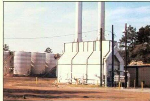
*Main heating system capable of 20 million BTU's per hour.*
