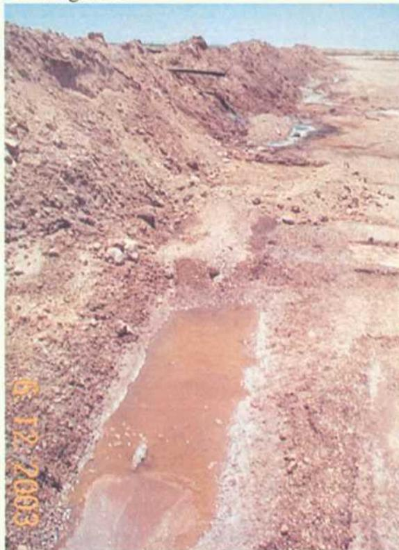
Photo 20. Solids evaporation Pit -7 and Pit 9 looking west. Fluids appear to be seeping from the pits.
