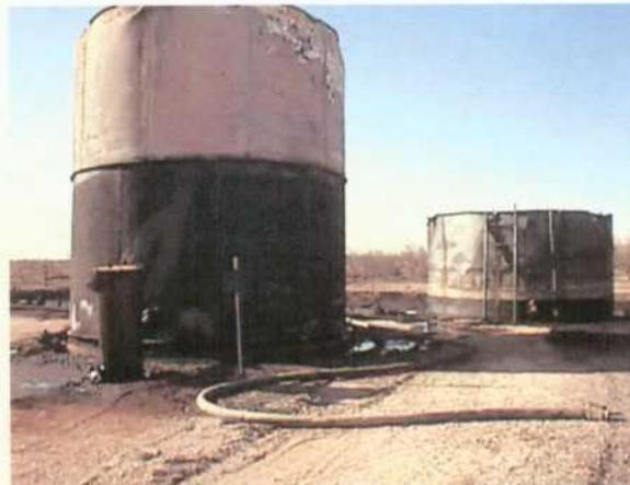
Photo 4: Tanks damaged from the fire. Tank on the left was half full and is still leaking.
