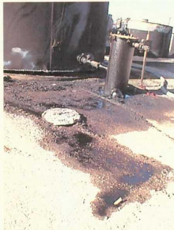
Photo 5: Oil on the ground still leaking from the tank.
