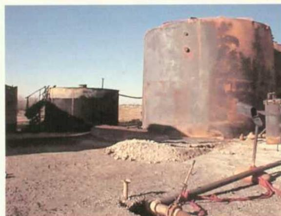
Photo 3: Tank blown off its bottom from explosion. Tank move 8 to 10 feet.
