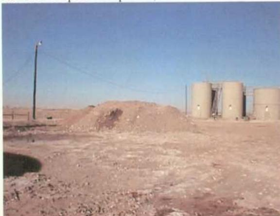
Photo 1: Treating plant untouched by the fire at the produced water receiving area. Pile of contaminated soil stockpiled for removal to CRI.
