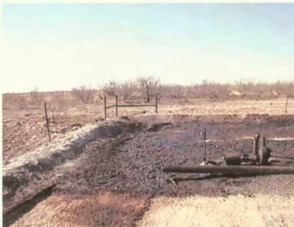
Photo 7: The southeast corner of the facility showing former berm height and fire damage well outside the fence line to the east and south.
