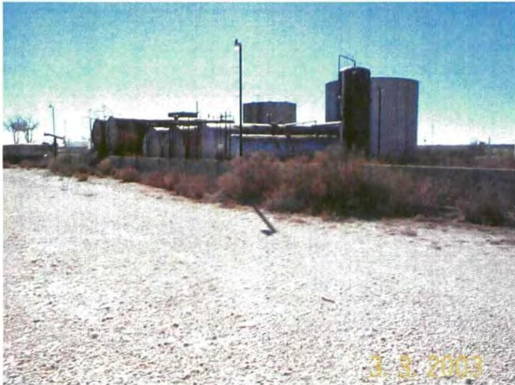
Photo 15: From left to right, 5 horizontal tanks, 1 vertical tank/separator, and two 3000 bbl tanks. Looking Southeast.
