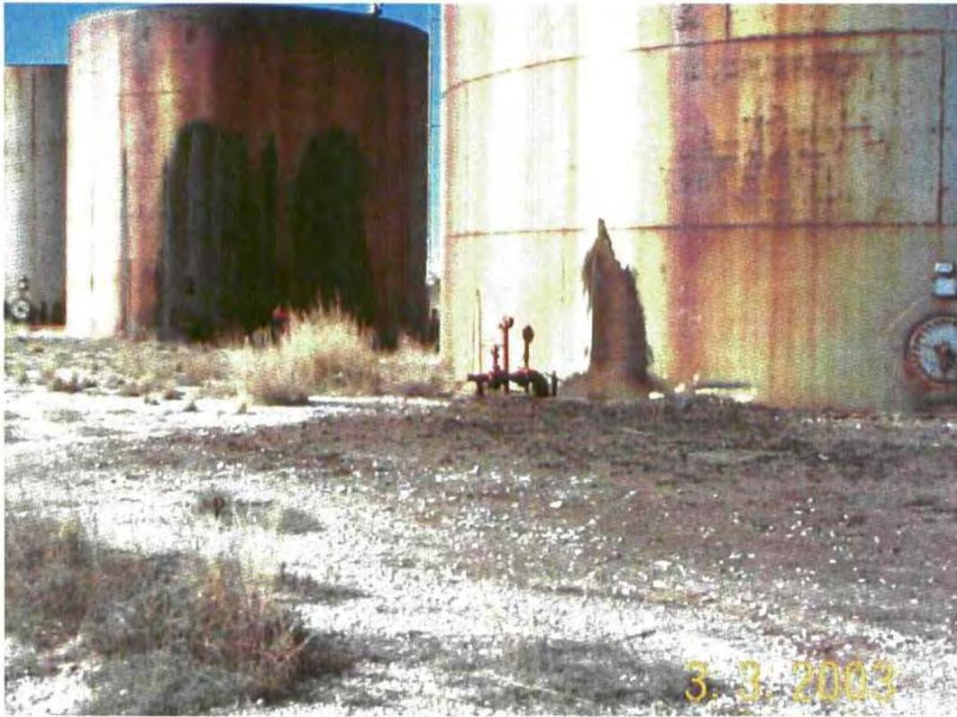
Photo 5: Leaking 500bbl tanks and 1000bbl tank. Looking south.
