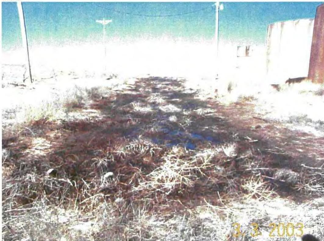
Photo 10: Pit/depression containing oil along south side of the row of 500 bbl tanks. Looking west.
