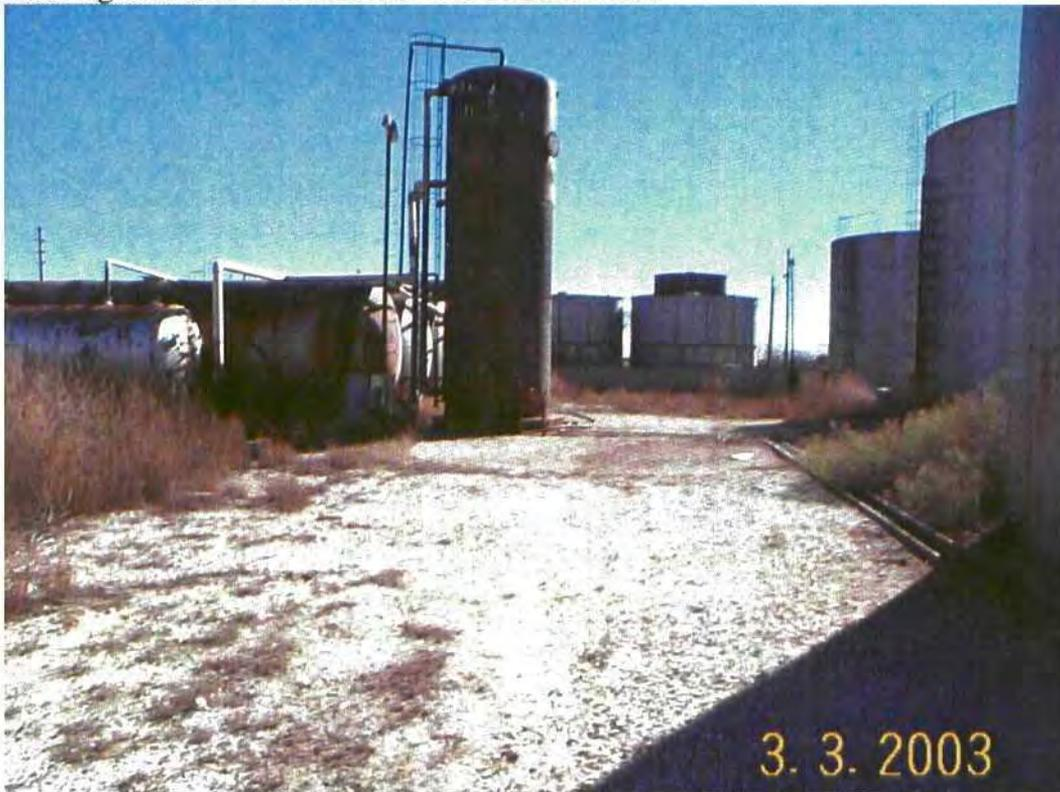
Photo 14: From left to right, 5-horizontal tanks, 1-vertical tank/separator, and 3-3000 bbl tanks on the right. Looking east.
