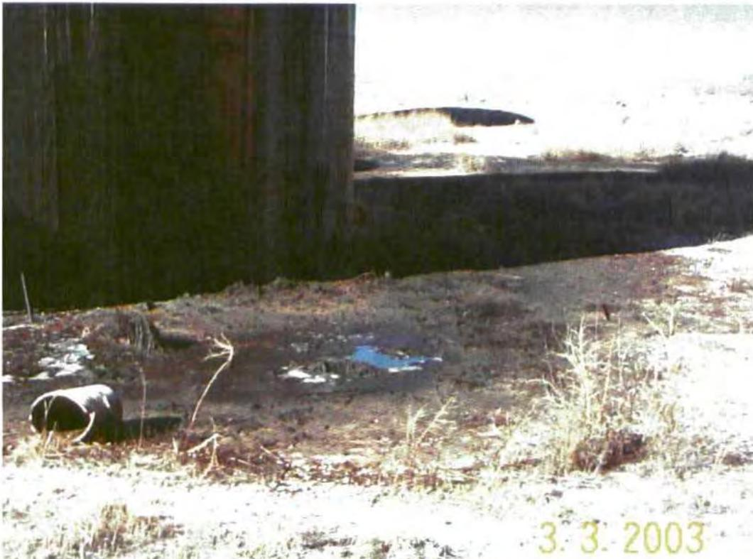
Photo 7: Contaminated soil surrounding the leaking 5000 bbl tank.
