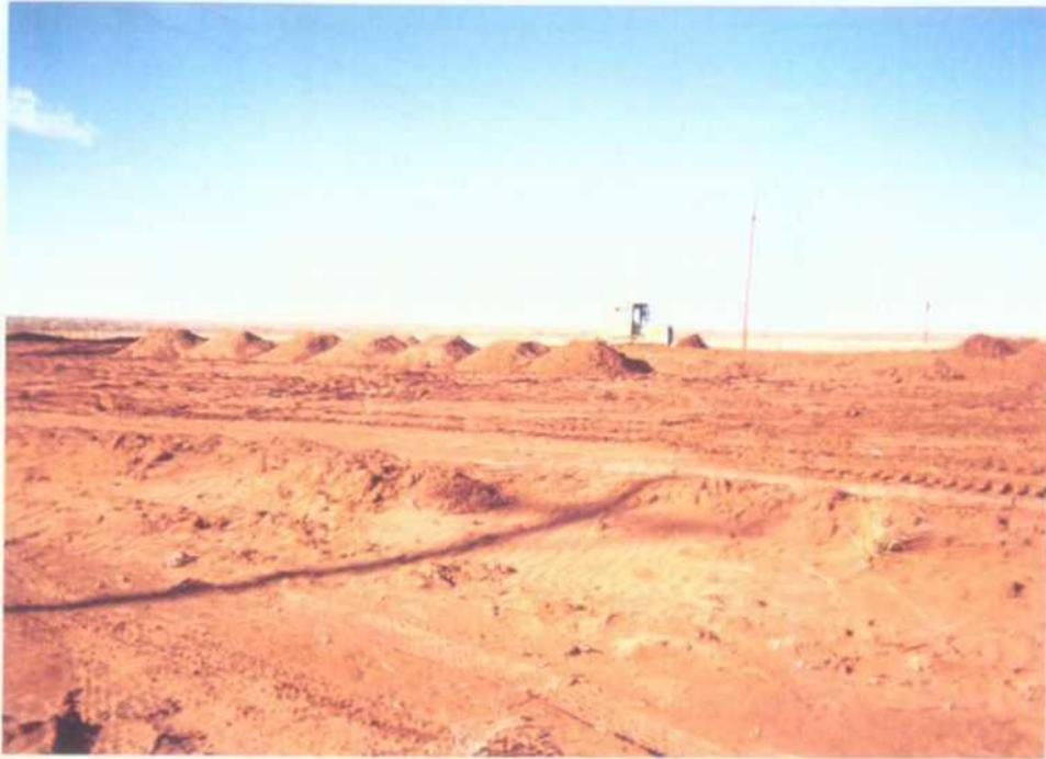
Photo 5: Placing clean soil over landfarm 2.
