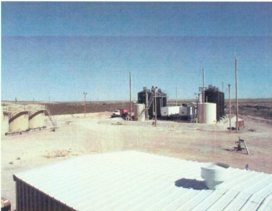
Photo 2: Yates produced water treatment facility at center. To the left are the treated, clean water tanks. Injection well is at the center right. Pump house roof in the foreground.
