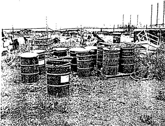
Drum storage area with "Selectox<sup>TM</sup> 33" on S side of plant violates drum secondary storage provisions of permit. No impermeable pad with curbing was present and empty drums are not stored on their sides (8-17-06)
