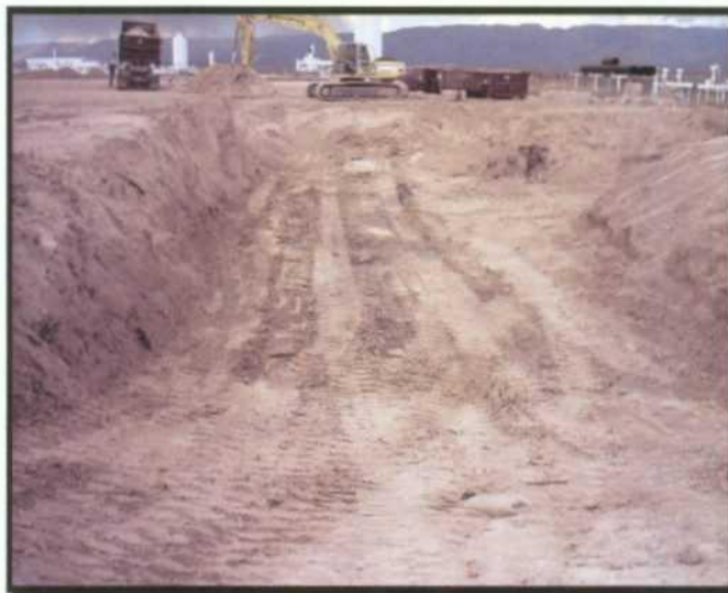
View to west showing excavation area
