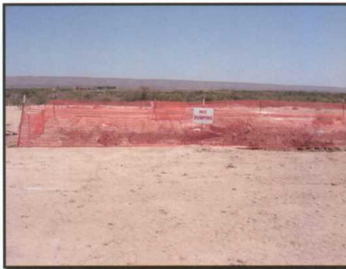
Pit excavation site control
