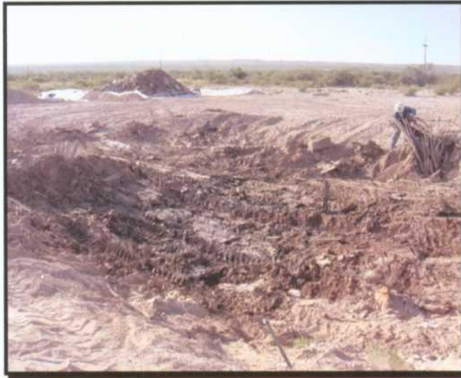
Pit excavation operation
