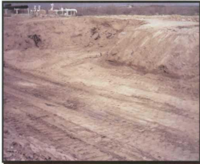
View to the northwest of completed excavation
