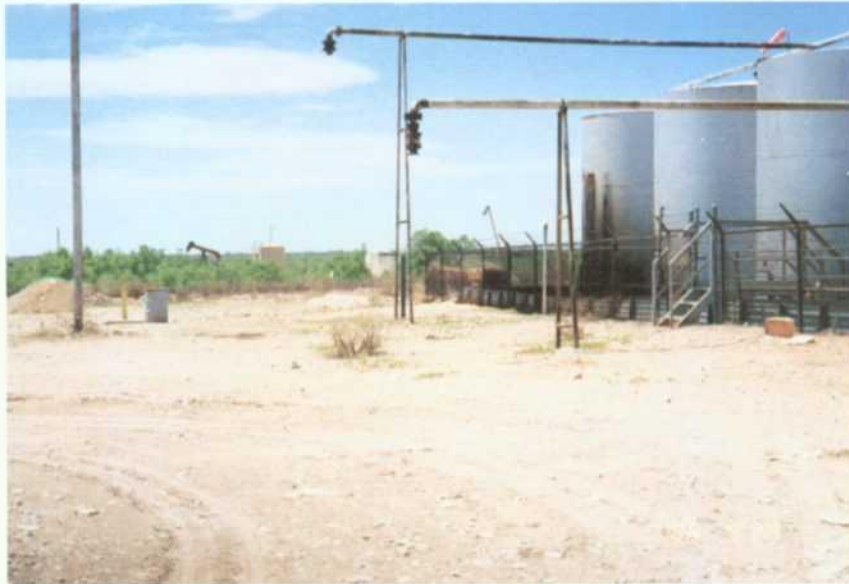
3. View to southwest of MW-3 and storage tanks.
