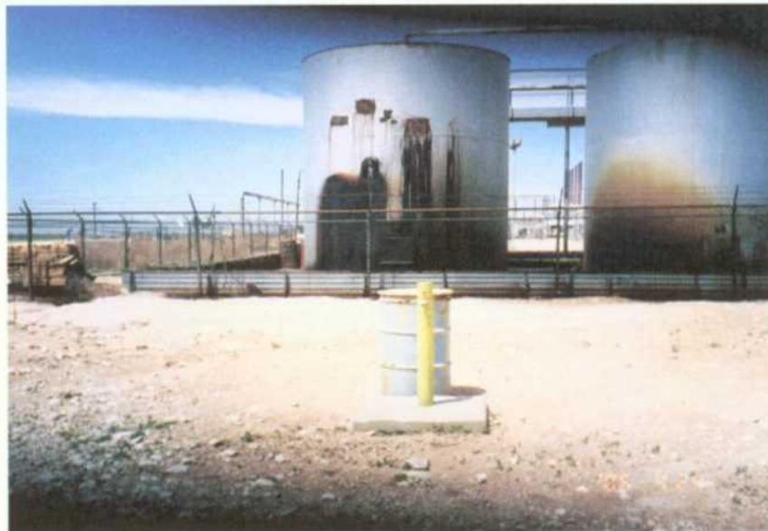
1. View to west of MW-3 and storage tanks.
