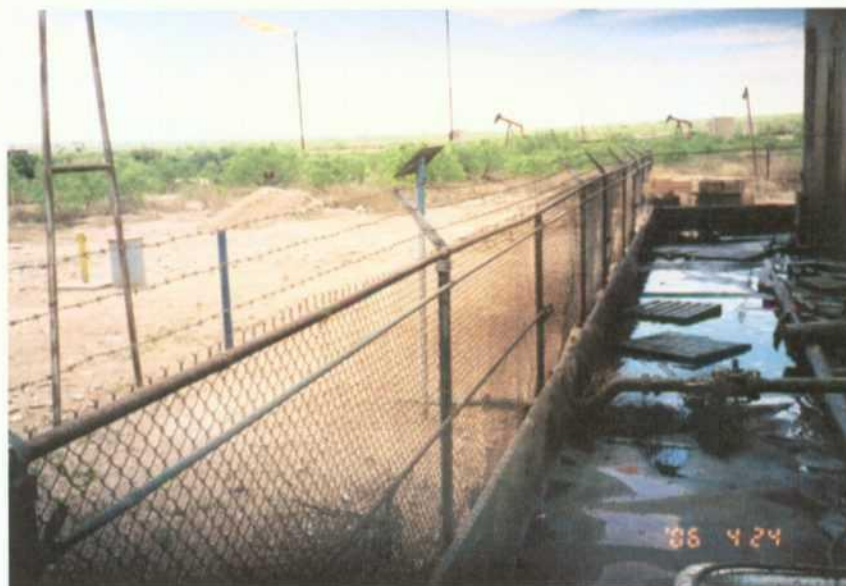
2. View to south of MW-3 and secondary containment of storage tanks.
