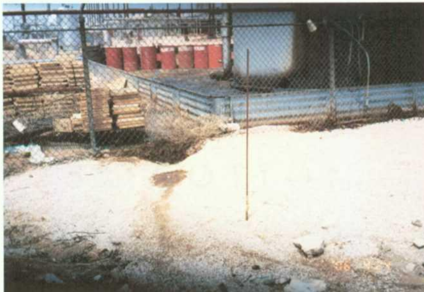
4. View to northwest of storage tank secondary containment near MW-3.
