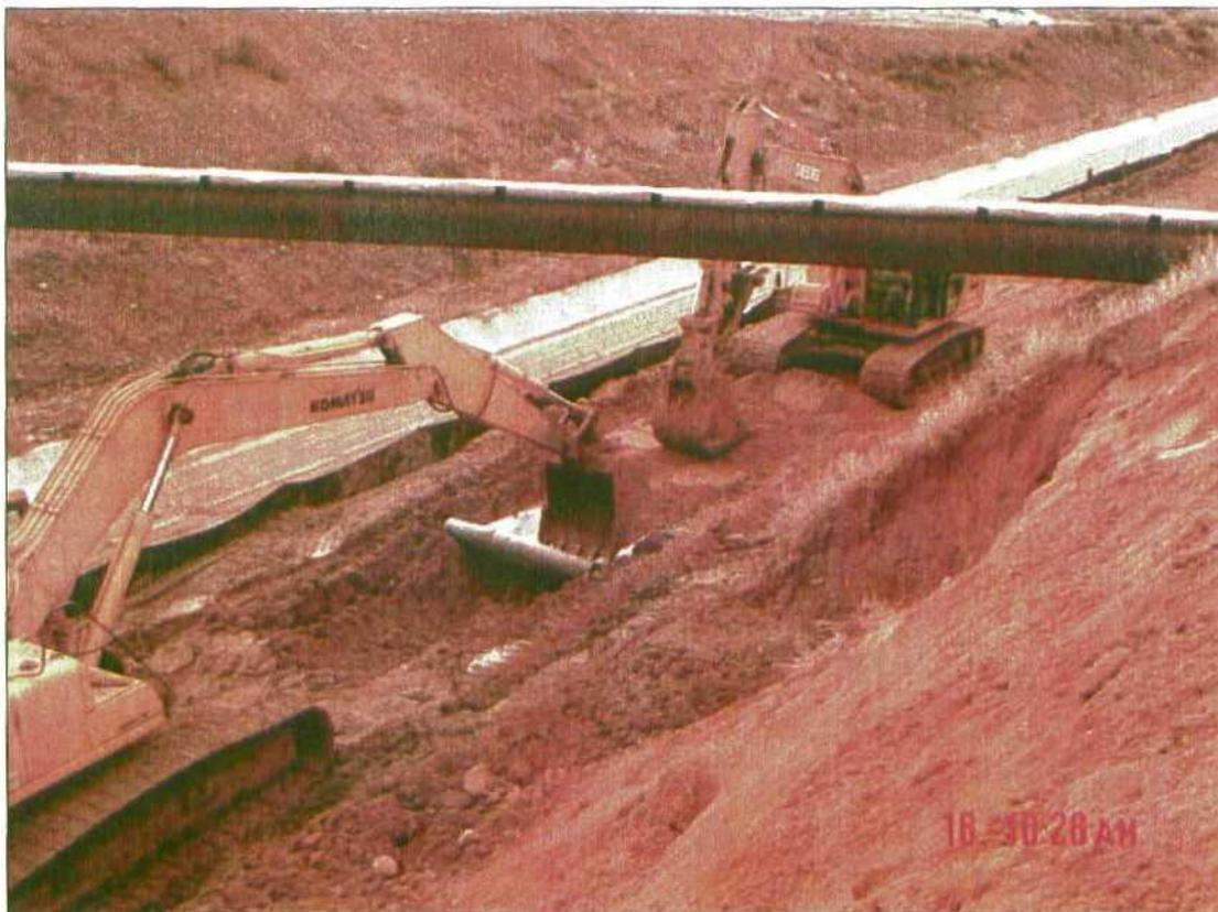
**Trench Capping Activities** – Approximately 3 feet of the trench backfill is removed for placement of the 7- 1/2 foot wide woven geotextile material. Bank-Run fill is placed over the geotextile material and leveled using the backhoe bucket.
