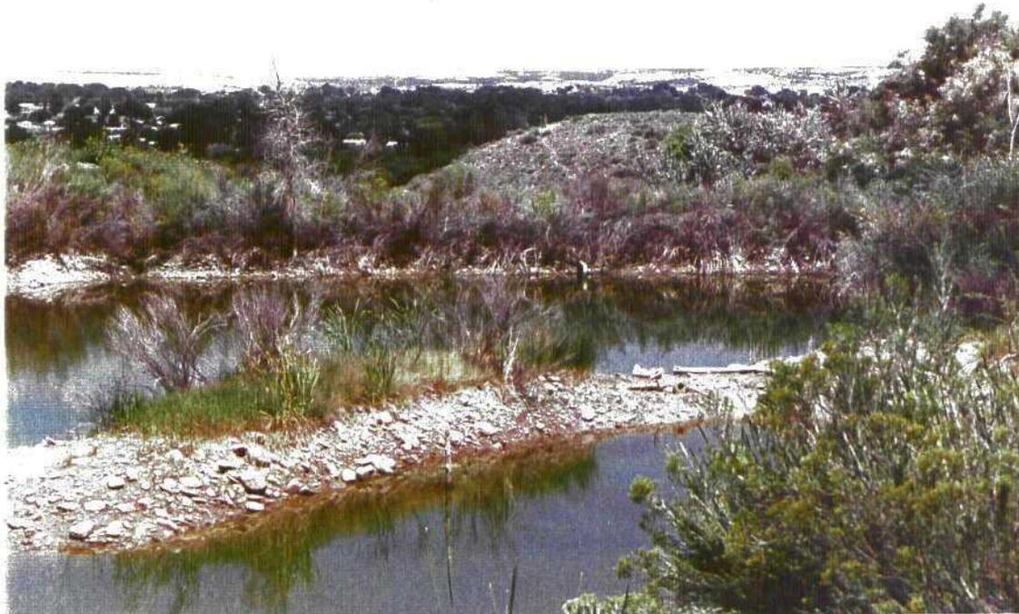
Upper of two, in series evaporation ponds which are the end of the waste stream from the main refinery waste water system. This pond discharges from a pipe (center left) to a lower pond.
