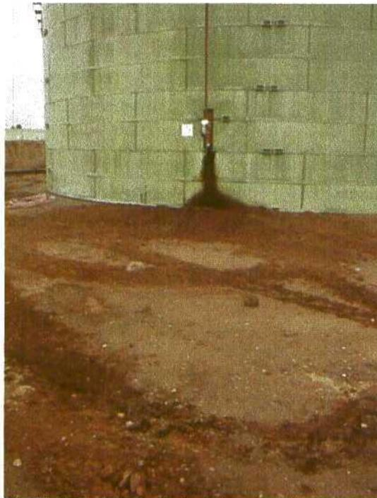
Pic 31-Tank#27 fuel oil tank gage leak and bioremediation area. Soils did not have any olfactory smells.
