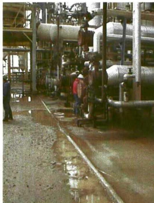
Pic9- Cat cracker area looking south. Picture shows pad and curb typical of all plant process areas.
