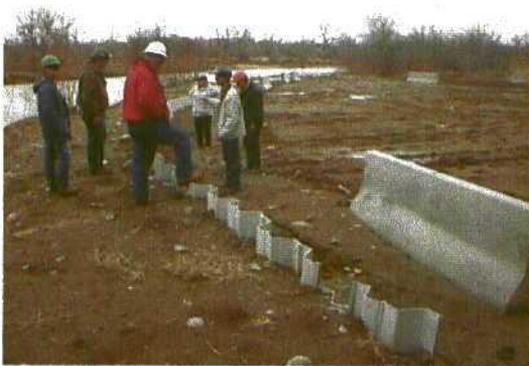
Pic22- Sheet piling and slurry wall installed next to the San Juan River to prevent hydrocarbons from seeping into river. Sheet piling is 11 feet deep, original design was to be 22 feet deep. Looking NE. upstream.
